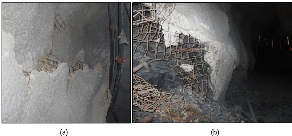
Figure 3 (a) Shoulder shear; (b) Buckled shotcrete rib
