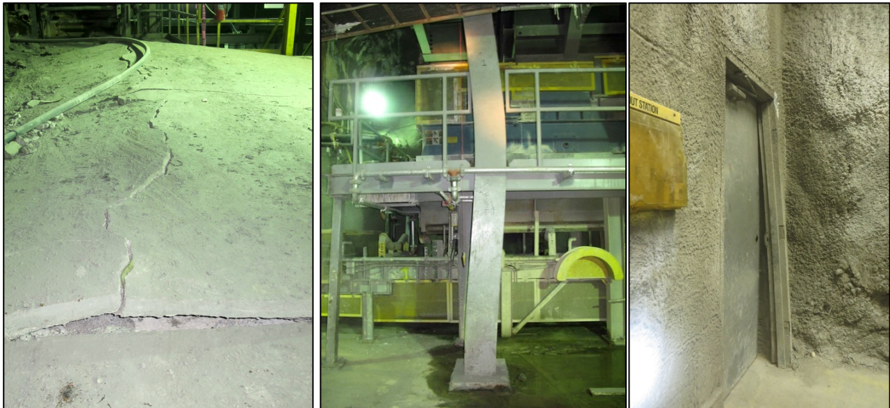
Figure 4 Infrastructure experiencing squeezing ground conditions, generally not tolerable
