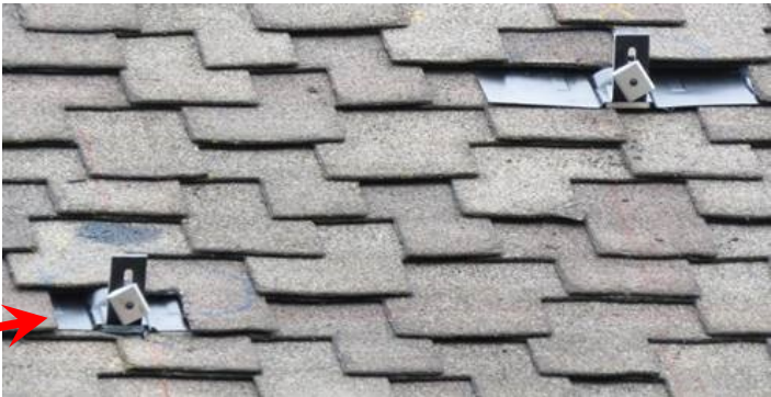
Fig. 2 Lifting up composite shingles to inset connection plates
