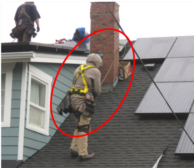
Fig. 4 This chimney obstructs the movement of the workers and reduces resistance capacity of the safety line
