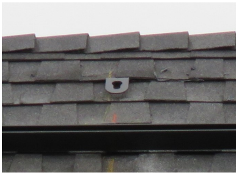
Fig. 10 This project installed Hitchclips along the roof ridge to serve as safety anchors.
