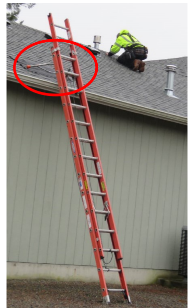
Fig. 14 Ladder with a ladder safety device
