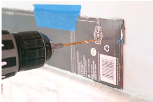
Towel Bar Installation Template (Brittany (2015). How to Install a Towel Bar Securely. www.prettyhandygirl.com/how-to-install-towel-bar-securely/ visited by Bardaweel on 1 NOV 2017)
