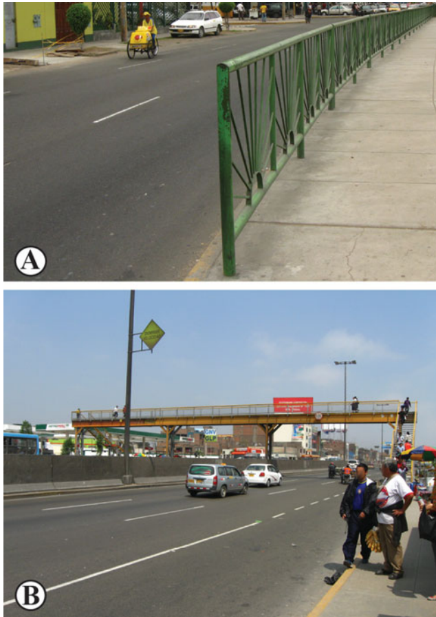
Fig. 3. (A) Example of a pedestrian barricade. (B) Example of a pedestrian bridge.
