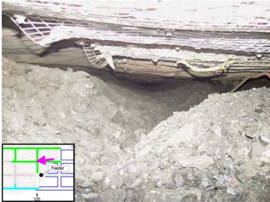
Figure 1.1: Crandall Canyon mine entry filled with rubble after the second failure incident
