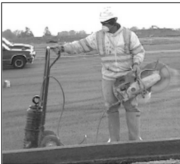
Figure 4. Cut-off Saw with Water Supply System for WSM.
