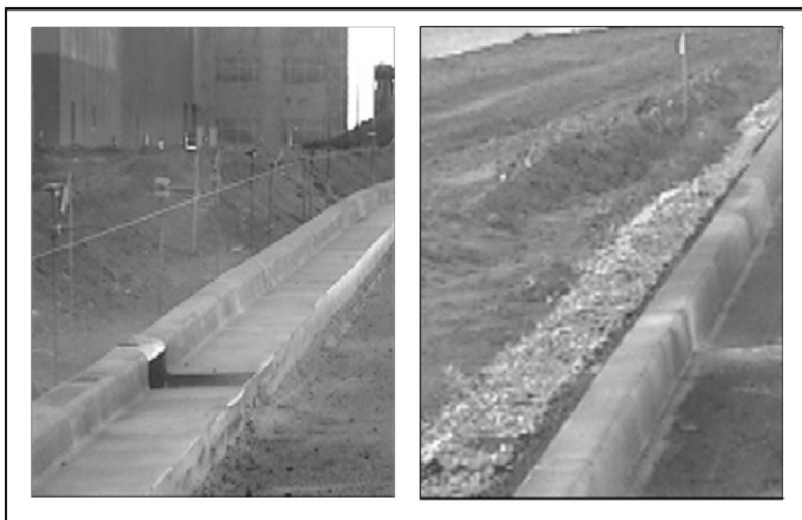
Figure 2. Chair Back Curb (on left) and Extruded Curb (on right).
