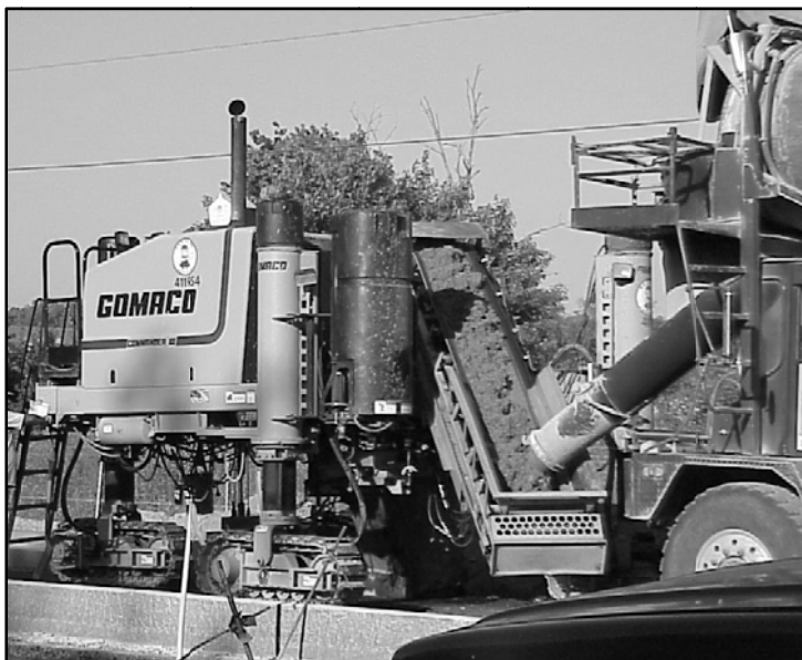
Figure 1. Concrete Curb Paving Operation.
