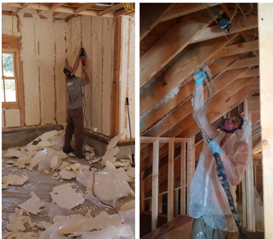
Figure 1. Photos of helper (left) and sprayer (right). The helpers cut and bundled freshly sprayed foam, sometimes without coveralls or gloves. The sprayer usually wore partial coverall, gloves, and an air-supplied respirator for protection from overspray.
