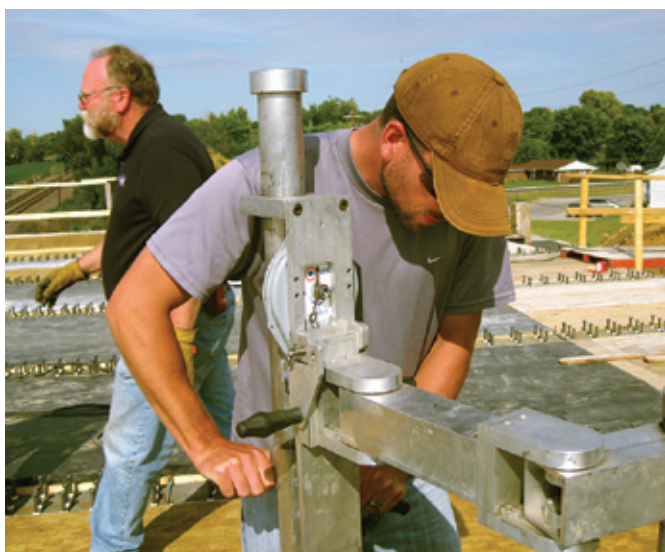
Dr. Fethke operates a prototype that enables workers to stand while stud welding. The tool's developer, a former ironworker, is in the background.
