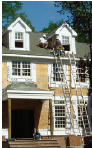
Typical New Jersey residential construction conditions faced by safety liaisons as recorded by project staff. Intervention can save the lives of workers at risk of a fatal fall.
