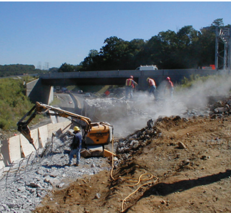
Silica dust and noise are a given on road construction and demolition sites. Dr. Woskie and her team seek protections through research.
