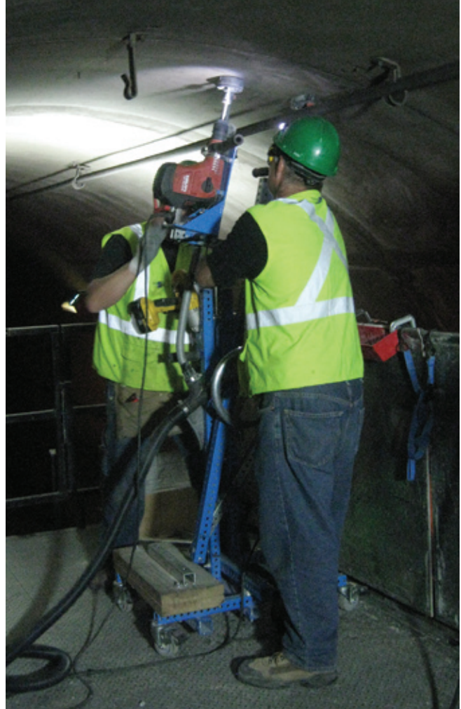
The Universal Drill Jig performed miles of overhead drilling, enabling the company to finish the project well ahead of schedule.
