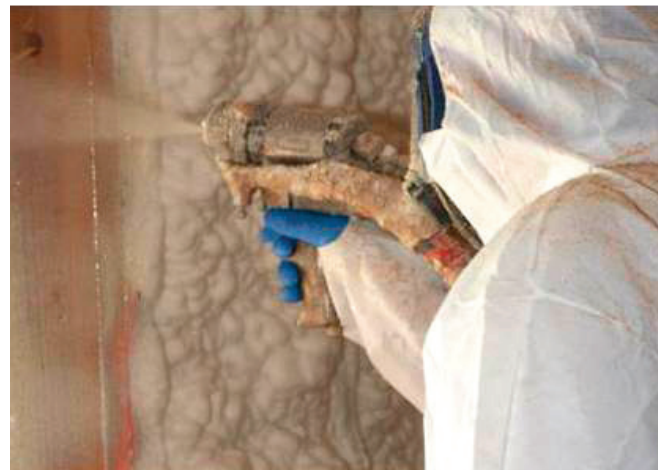
Proper protection from isocyanates in spray-foam insulation can prevent work-related asthma.
