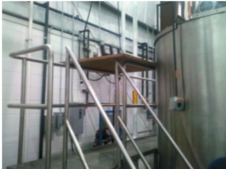
After OSHA 10-hour training, Apprentice Greg Chrisman refused to work on this jerry-built scaffold. The union stepped in to fix the unsafe condition; Chrisman received a commendation.
