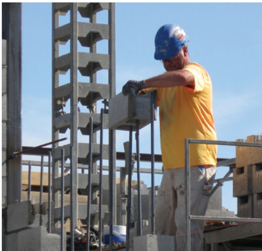
Lifting and laying block over rebar
