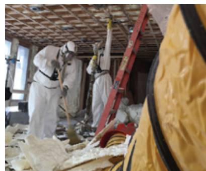
SPF insulation: spraying, trimming, and cleanup
