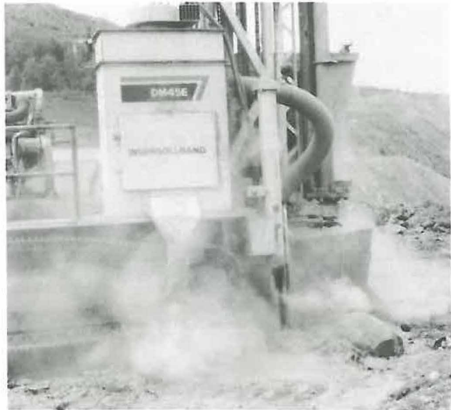
Figure 2. Typical dusty atmosphere created by rock drilling operations.
