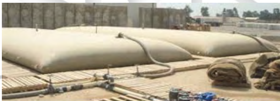
Water bladders and distribution
