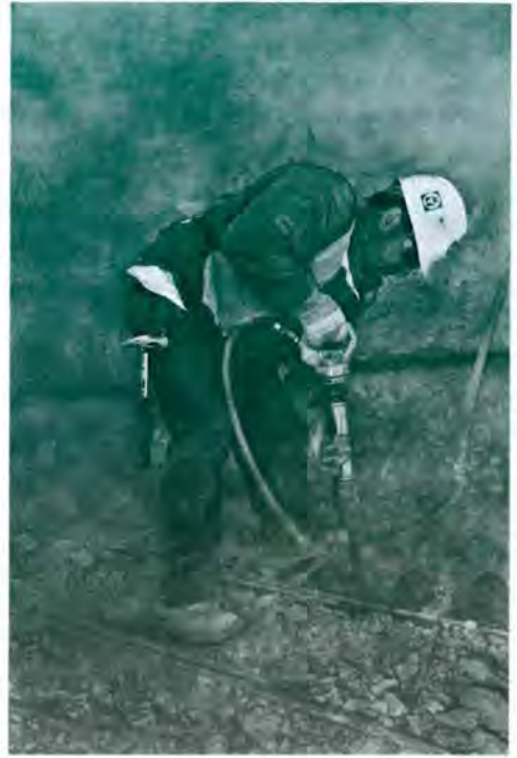
Figure 12A-4. Improper and proper hearing protection: (A) Cotton earplugs are ineffective in protecting a worker from loud noise. (B) This jackhammer operator is appropriately wearing earplugs. (Photographs by Earl Dotter.)
