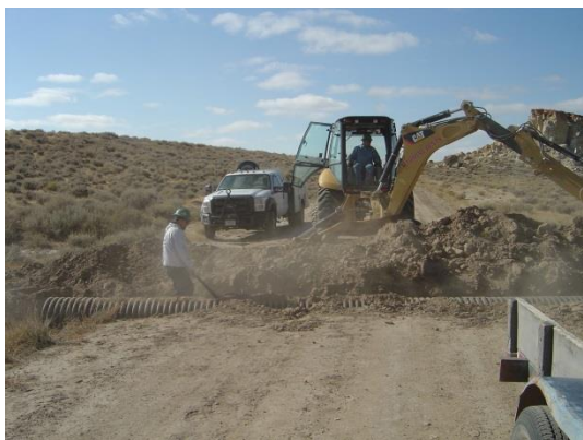
Figure 1. Backhoe in use during culvert replacement.
