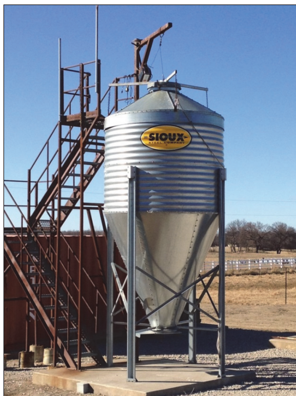
Figure 1. The 1.83 m (6 ft) diameter steel bin used during measurement of entrapment pressures.
