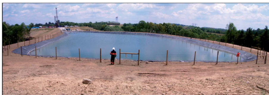
Fig. 4 Hill top pit incised into subgrade with geomembrane liner.
