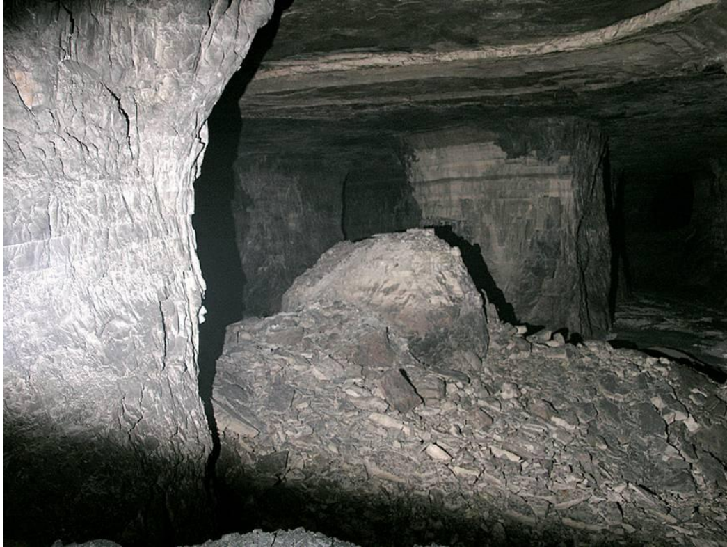
Figure 6. Remaining stump of a collapsed pillar in an abandoned area.
