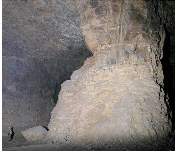
Figure 14. Rib failure related to large, angular discontinuities adjacent to a fault zone.
