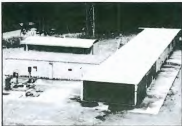
Fire suppression facility
