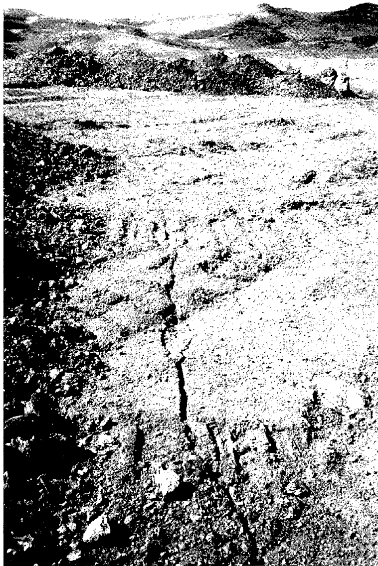
Tension cracks (above) and water seepage (right, as indicated by researcher) can be indicators of potential slope failure
