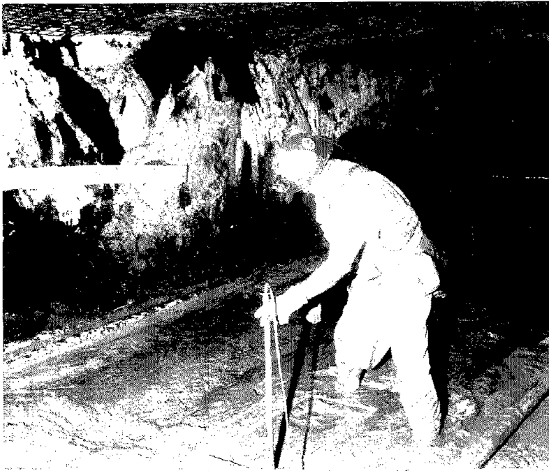
Earth pressure cells and strain gauges being installed to monitor the stability of backfill
