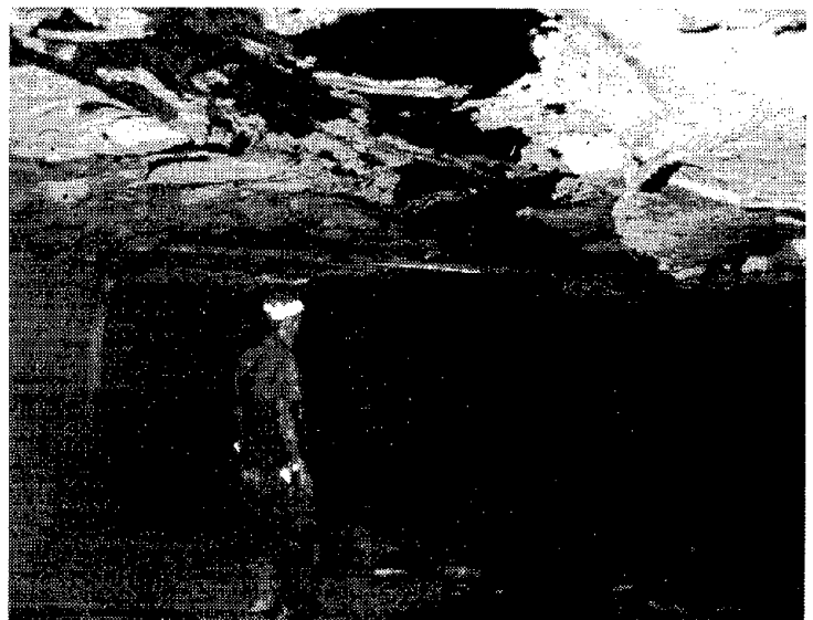
Roof fall caused by failure of roof support system
