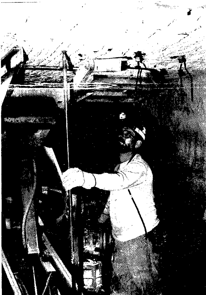
Installing roof bolts is the most hazardous job in an underground mine.
