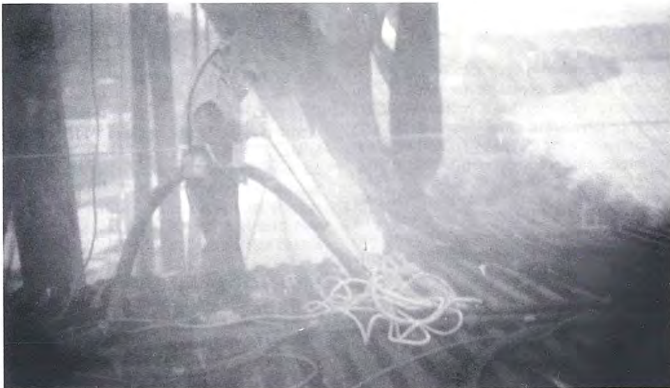
Figure 1. Construction worker using a HEPA-filter vacuum inside a containment structure. Note that the worker is obscured by a high airborne concentration of dust.
