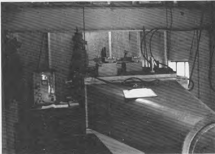
Figure 13. Electrostatic Precipitator installed for testing showing ductwork.
