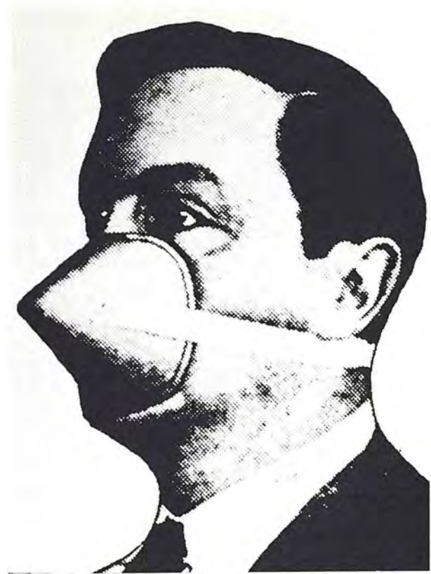
Figure 2-7. Pulmosan dust mask, ca 1920. Very similar to single use dust respirator used today.
