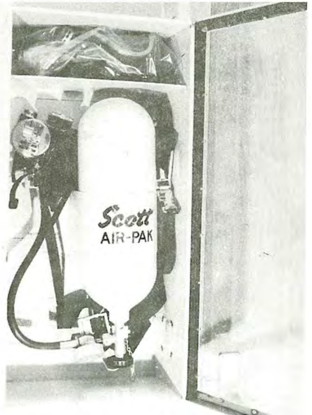
Figure 9-6. Wall-mounted storage cabinet for a SCBA.
