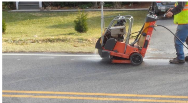
Figure 38. Nellies Cave Road Repair
