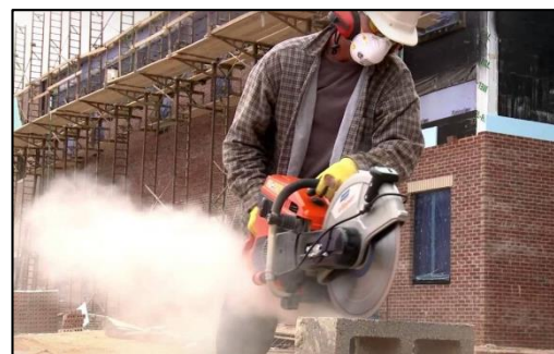
Figure 1. Handheld cut-off saw producing dust containing silica
