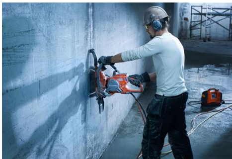
Figure 41. Husqvarna K6500 Power Cutter: Allowing Full Blade Depth Cut
