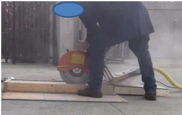
Figure 80. Guiding Rod Test With Back of LEV Lifting
