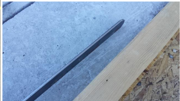
Figure 89. Metal Ski Design Scratching Concrete
