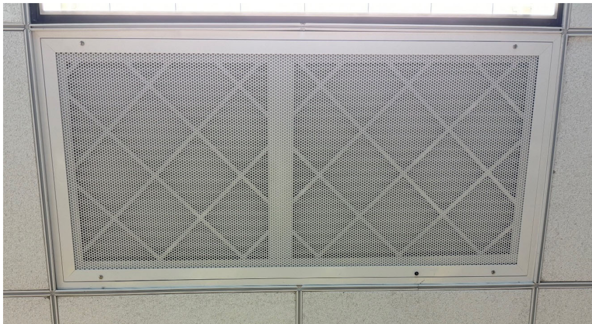
Figure S3: Air return and HEPA filter.
