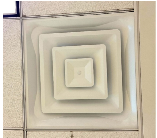
Figure S2: Square cone air supply diffuser.
