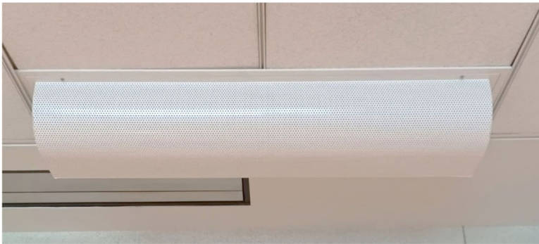
Figure S1: Radial air supply diffuser.
