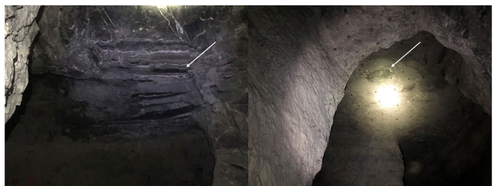
Fig. 4 (Left) Breakage to bedding planes noted in the measurement area. (Right) Small roof failure due to bedding separation in an area where the number 55 thin shale marker bed is in the immediate roof section
