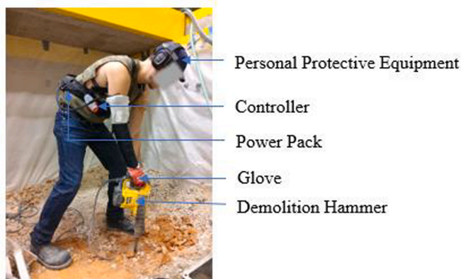
Fig. 4. The H-EXO (Ironhand 2.0) used for breaking concrete.
