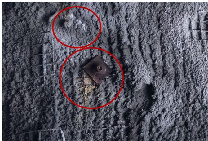
Figure 2.1.2. Signs of water precipitation on the walls at the SX To classify the instabilities at the new decline, we used the classification method proposed by Kaoutar Clero et al, in 2020, to ease the determination of the monitored parameter. While classifying geotechnical instabilities,
