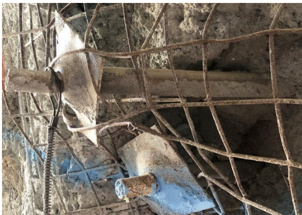
Figure 1.2.3. Image of expansion bolts after expansion with water pressure and 3'x3' mesh near portal at the SX
