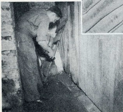
LEFT — Adjunct of Basement Floor and Wall is Inspected.
