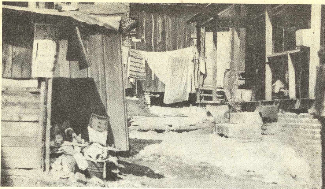
Trash and sheds in this yard not only constitute fire hazards but also leave little space for children to play.
