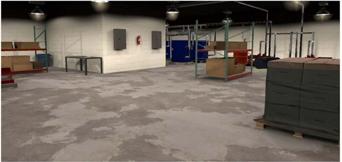
Figure 1. Machine room environment
