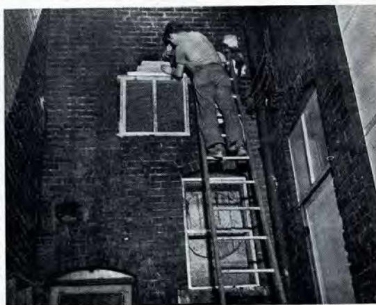
Installing ratproof screens and pointing up brick around windows in building in Chattanooga.
