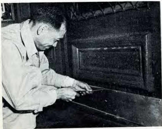
Trainee installing a metal plate as a rat-proofing measure.
