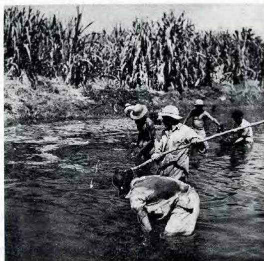
Removing aquatic vegetation from drainage ditch at Ft. Buchanan.
