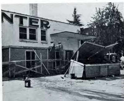
Building a ratproof garbage stand back of a large food market. Note dilapidated wooden garbage stand previously used.
