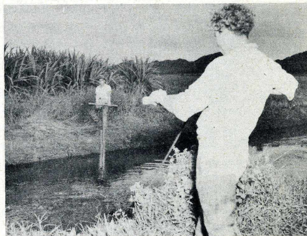
Ditch Clearing Device in Operation
