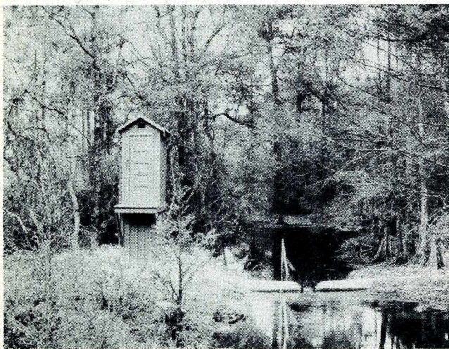
Gage House and V-notch Wier
