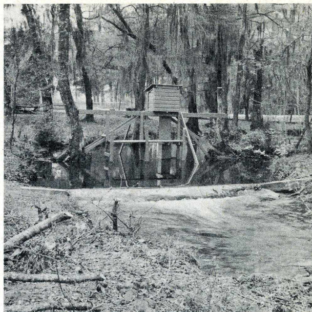
Recorder Shelter and Artificial Control
