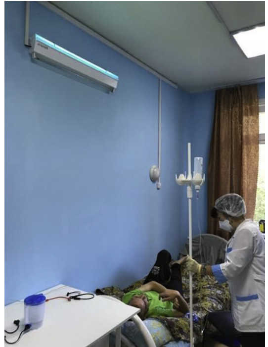
Fig. 5. Upper-room GUV fixture in use in a Russian hospital.
