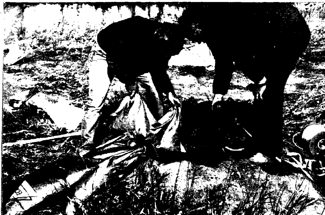
FIGURE 5-4: THE LOADING OF ANFO INTO A BLASTHOLE WITH THE BLASTING TAPE BEING USED TO MONITOR THE COLUMN RISE
