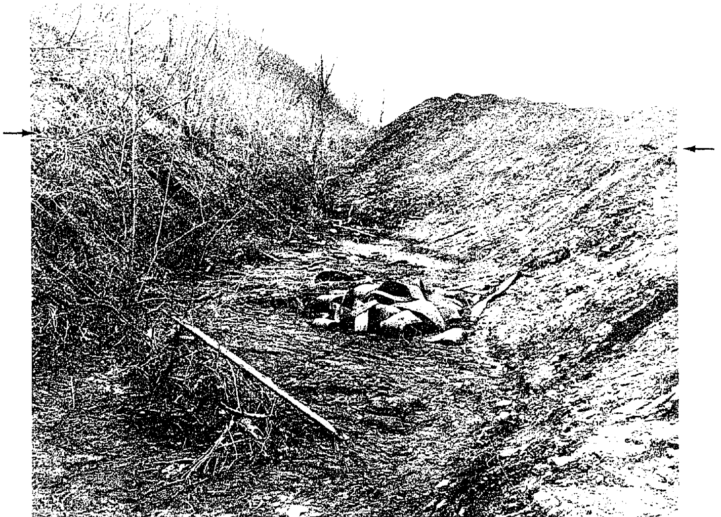
HIGH WATER LINE (ARROWS) AT APPROXIMATELY ELEVATION 1709 AT LEFT SIDE OF REFUSE BANK PHOTO TAKEN ON FEBRUARY 29, 1973
