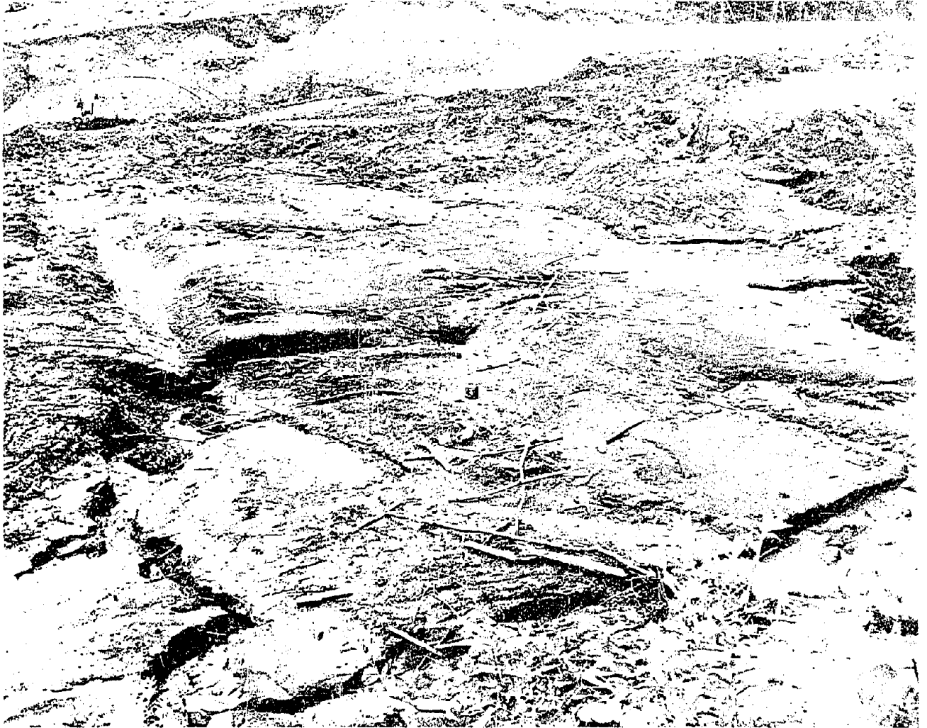
PORTION OF THE "ROLLED AREA" OF TRANSLATED POOL 2 SLUDGE. THE SMOOTH, FLAT AREA IS ONE OF THE MAJOR BLOCKS OF SLUDGE THAT WERE MOVED AS UNITS DURING THE FAILURE.
