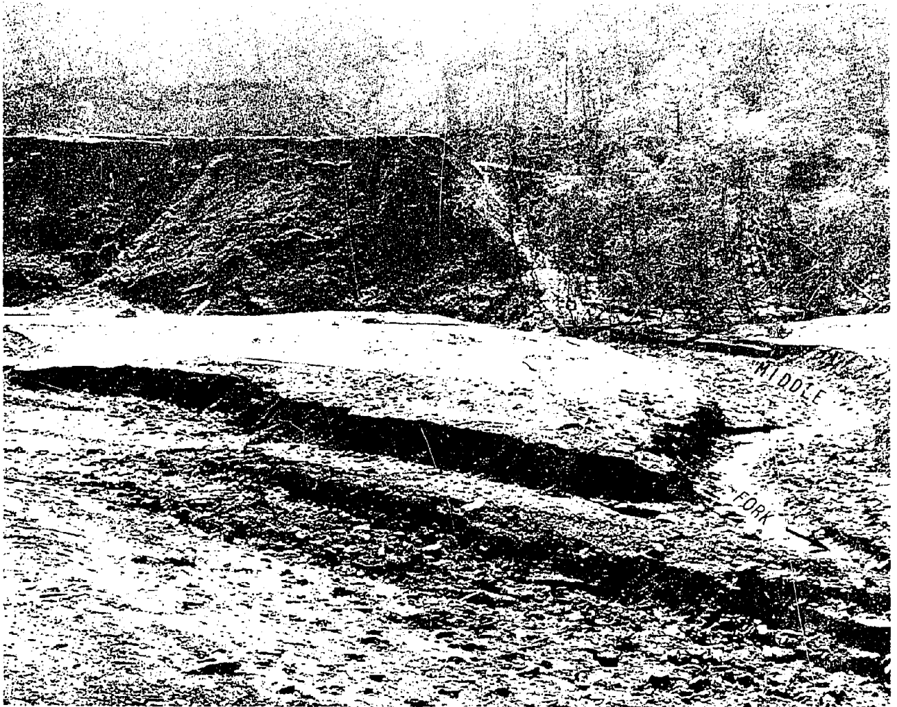
DOWNSTREAM PORTION OF LEFT ABUTMENT REMNANT OF DAM NO. 3, FEBRUARY 29, 1972. THE LOW, SCoured MOUND IN THE CENTER EXTENDED TO THE RIGHT DURING THE FIRST STAGES OF THE FAILURE. IN THE FINAL EMPTYING OF POOL 3, THE MOUND WAS DISECTED BY MIDDLE FORK AS SEEN HERE.
