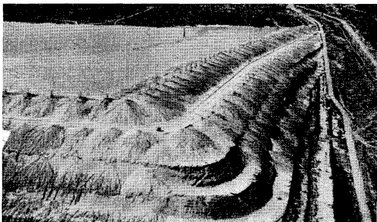
PHOTO A. VIEW SHOWING CONES OF TAILINGS DEPOSITED AROUND INDIVIDUAL CYCLONES AT SAN MANUEL, ARIZONA. NOTE NUMBER AND SPACING OF CYCLONES.
