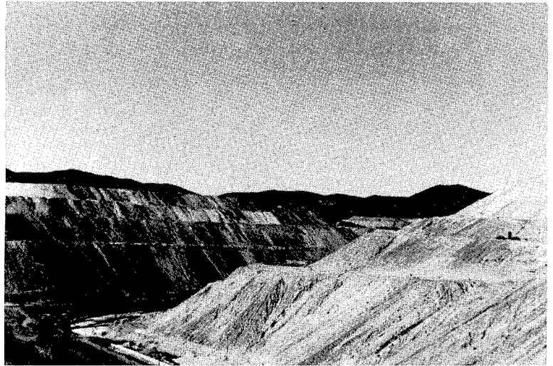
PHOTO B. MAIN EMBANKMENTS AT CHINO LEACH DUMP. NOTE THE DRILL RIG ON BENCH TO THE RIGHT.
