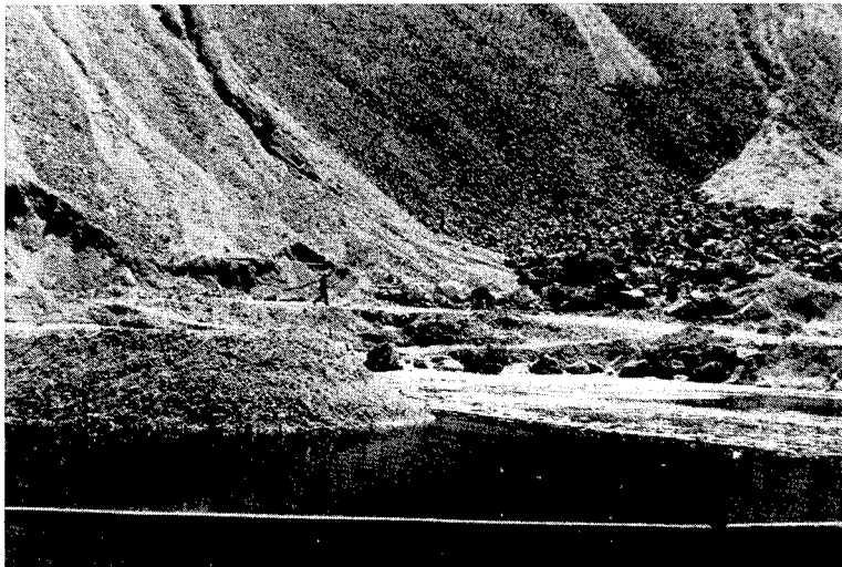
PHOTO C. TOE OF DUMP IN FOREGROUND OF PHOTO B. NOTE BOTH THE COLLECTION OF ACID SOLUTION AND MAN IN FOREGROUND FOR SCALE.
