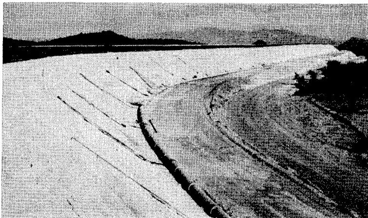
PHOTO A. TRANSITE HEADER WITH PARTIALLY BURIED LATERALS AT THE SILVER BELL UNIT OF THE AMERICAN SMELTING AND REFINING COMPANY, ARIZONA.
