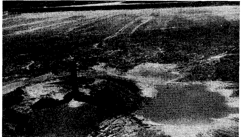
PHOTO D. AERIAL VIEW SHOWING REINFORCED CONCRETE DECANT TOWER AT MORENCI, ARIZONA.
