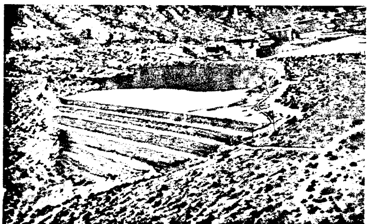
The above photographs depict various elements of mill tailings disposal. UPPER LEFT, Tailings dam being constructed by typical upstream method; UPPER RIGHT, Tailings being discharged by peripheral spigotting; LOWER LEFT, Tailings being discharged by hydro-separators (cyclones); LOWER RIGHT, Completed tailings dam.
