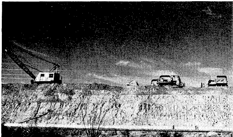
PHOTO C. DOZER AND SHEEPSFOOT ROLLER COMPACTING RAISED EMBANKMENT.
