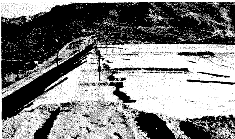
PHOTO C. THE NEW TAILINGS DEPOSIT AT SUPERIOR, ARIZONA SHOWING PITS EXCAVATED TO OBTAIN MATERIAL FOR HAND-BUILT DIKE AT EDGE OF DEPOSIT IN LEFT PORTION OF PHOTO. STEEL LATERAL PIPES PARTIALLY OBSCURE THE DIKE ITSELF. THE DEPOSIT IS NOW READY TO RECEIVE ANOTHER RAISE.
