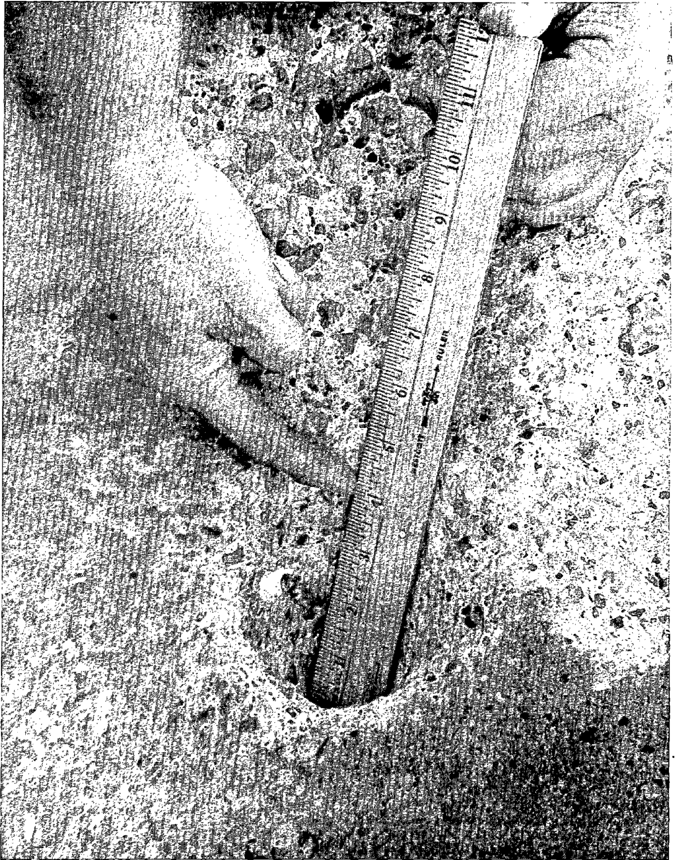
FIGURE 6-1. SINGLE-SHOT DAMAGE TO CONCRETE WITH NOZZLE STATIONARY; TEST R-43
