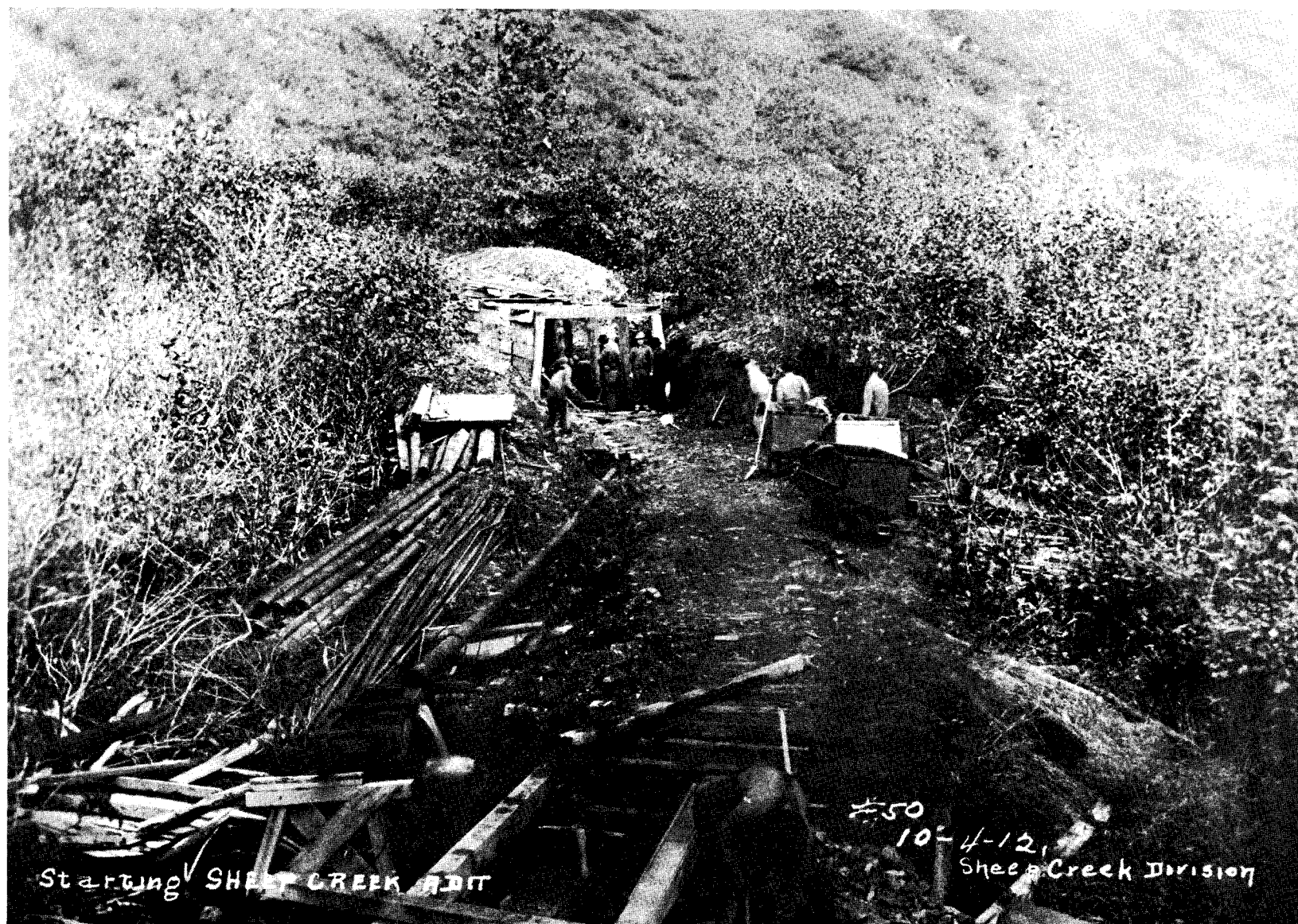
Figure 18. Beginning the 10,400 ft-long Sheep Creek Tunnel in 1912 which would connect with the Perseverance mine (Winter & Pond Coll., Alaska Historical Lib.)
