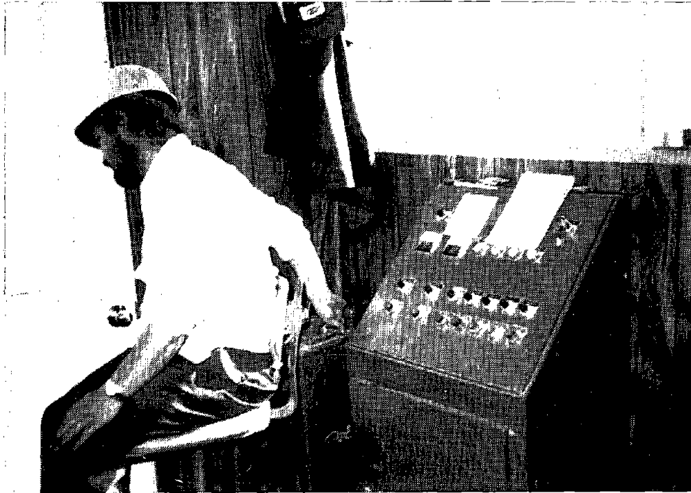
FIGURE 51. - Plant B - primary crusher control booth.
