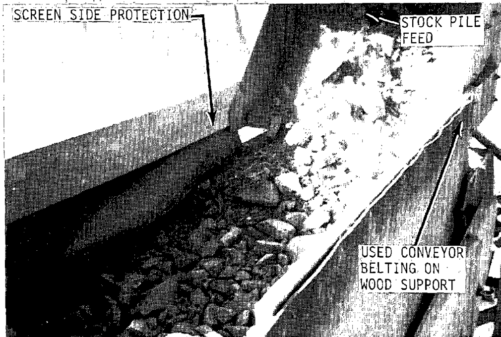
FIGURE 33. - Plant A screen side protection.
