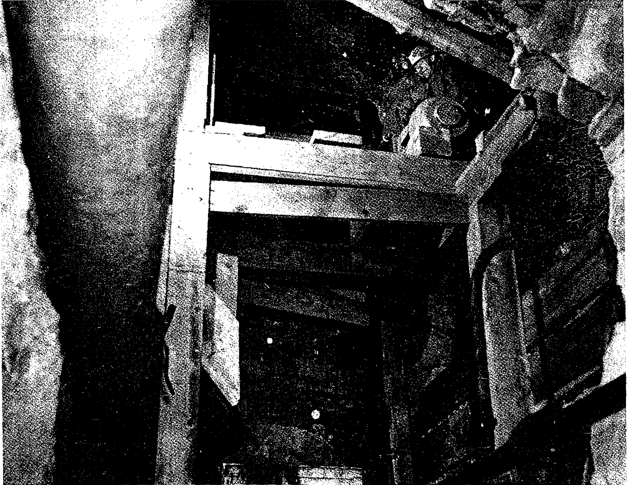
FIGURE 15. - Filling Mine Car at Scraper Chute in Mineral Joe Mine.
