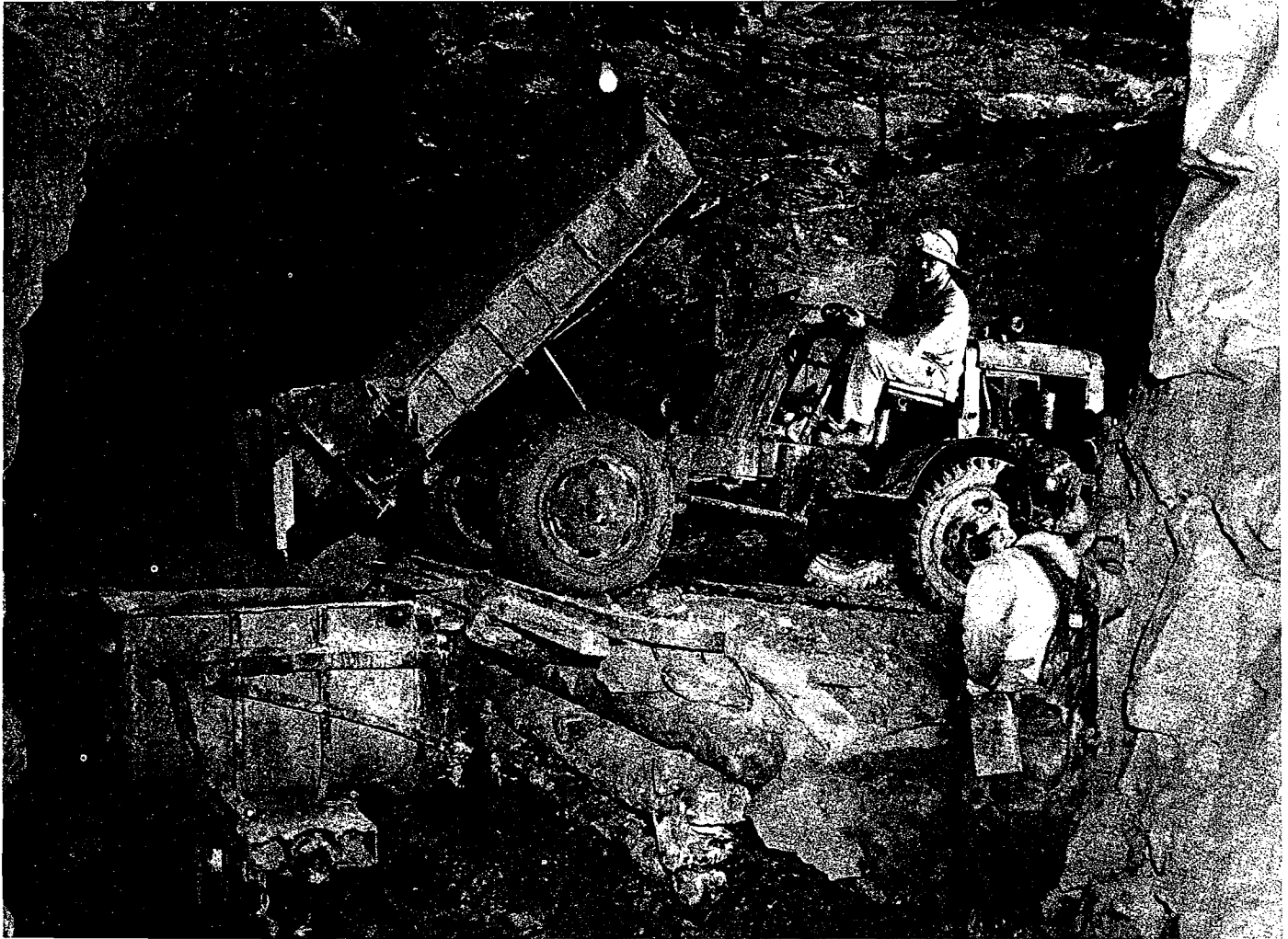
FIGURE 6. - Dumping Load Into Hoisting Car at Main G-1 Incline.
