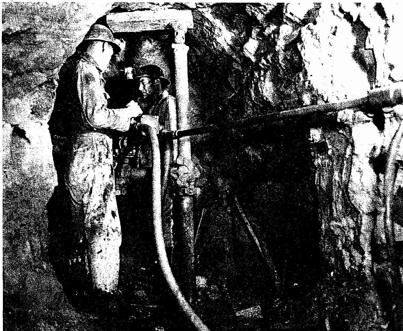
FIGURE 22. - Testing Ahead With Underground Diamond Drill.
