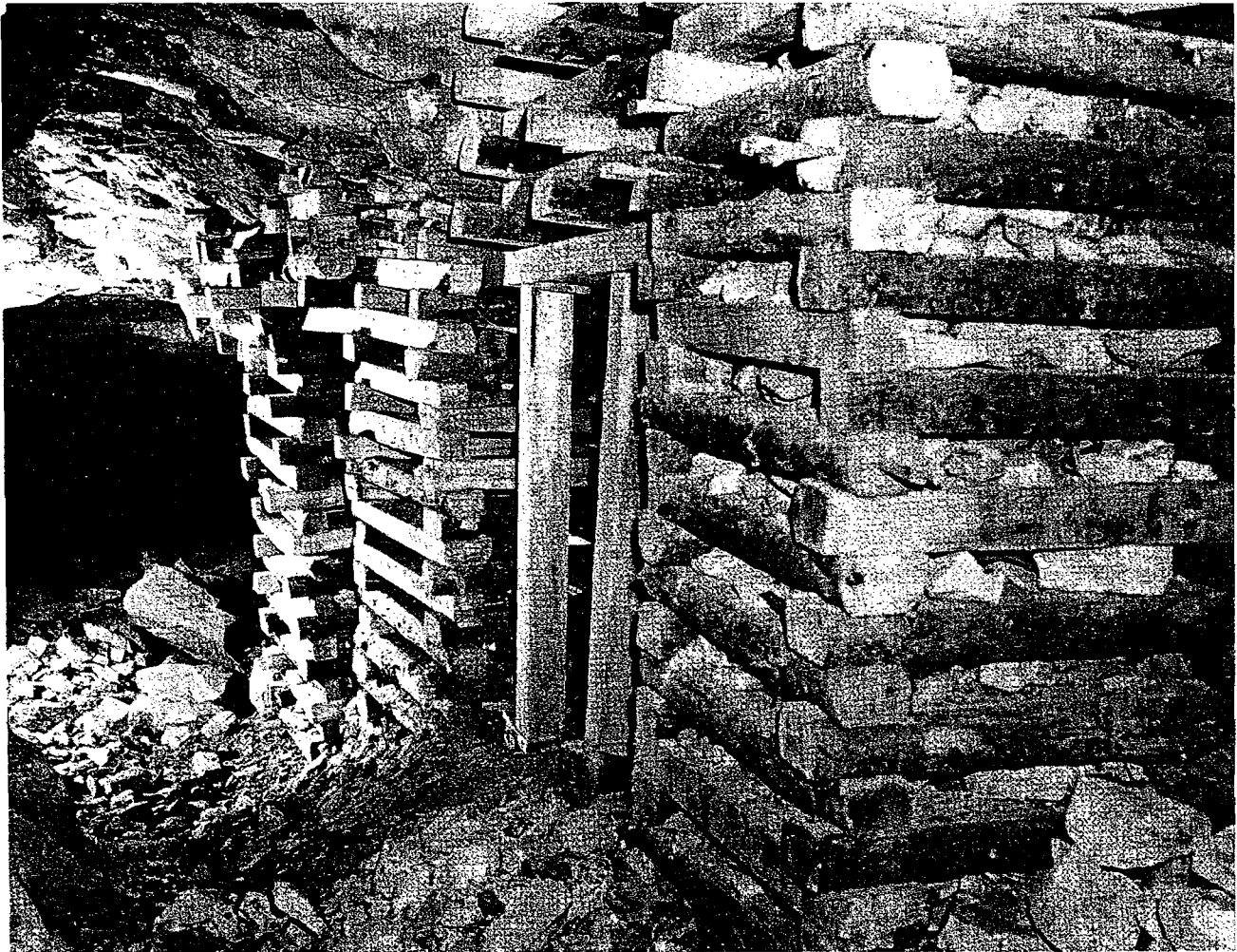
FIGURE 16. - Row of Cribs Near Caved Stope in Mineral Joe Mine.
