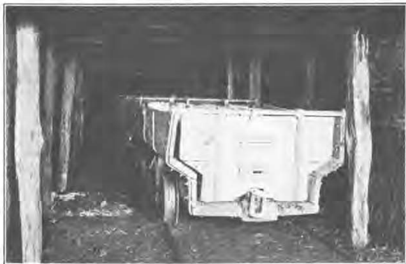
FIGURE 31.—Trip of cars used in timbered section in pressure-loss tests
