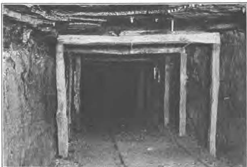
FIGURE 22.—Split-timber sets used in pressure-loss tests
