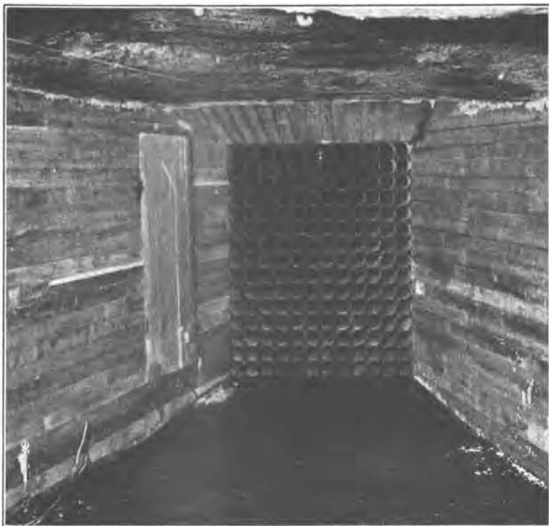
FIGURE 8.—Approach side of 1B-100 air-measuring station
