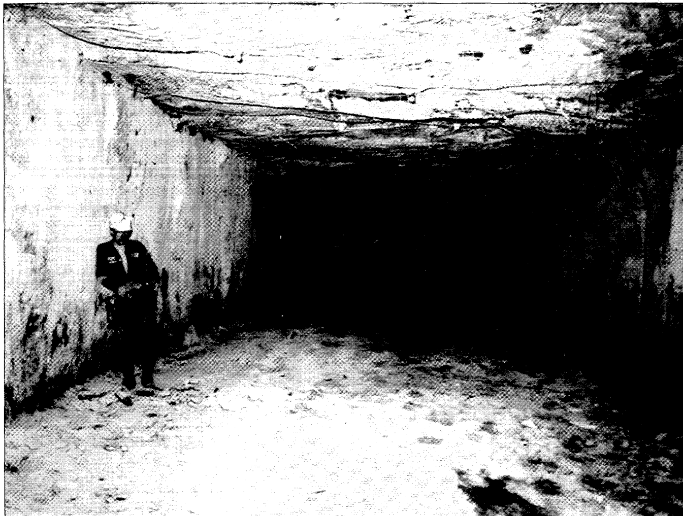
Bleeder entry in Castle Gate No. 5 Mine. Intact, unfractured ribs and minimal rib sloughage are typical of these workings. "D" Seam height, approximately 3 m (10 ft), is indicated by mine engineer beside rib.
