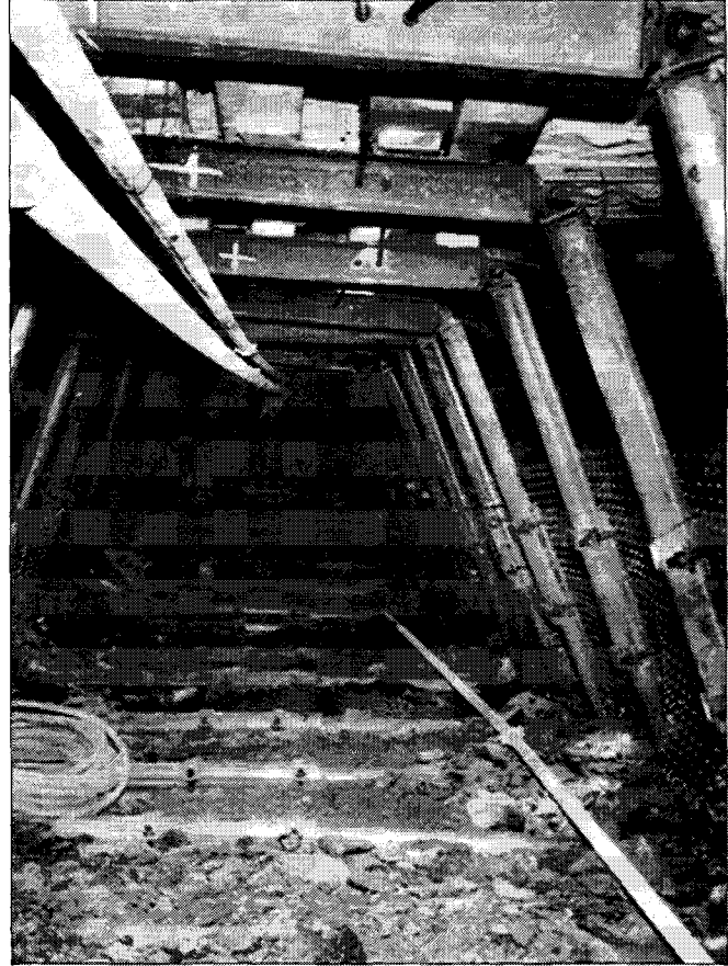
Yieldable steel sets in 5th Left gate road. In subsequent gate roads, this expensive secondary support system was abandoned in favor of conventional wooden cribbing.
