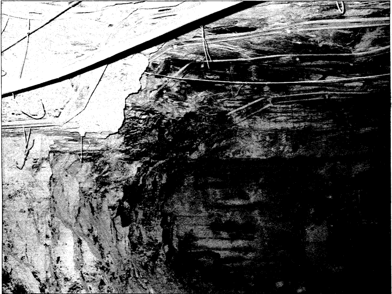
Domed roof fall area in Sunnyside No. 1 Mine near gate road study area. Besides poor roof conditions, horizontal stresses often contribute to occurrence of domed falls.
