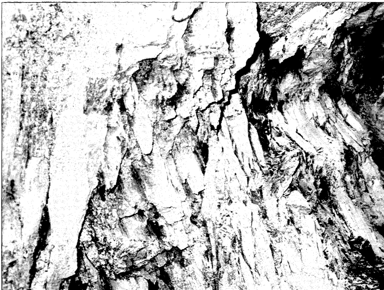
Yielded gate road panel rib in northeast part of Sunnyside No. 1 Mine.
