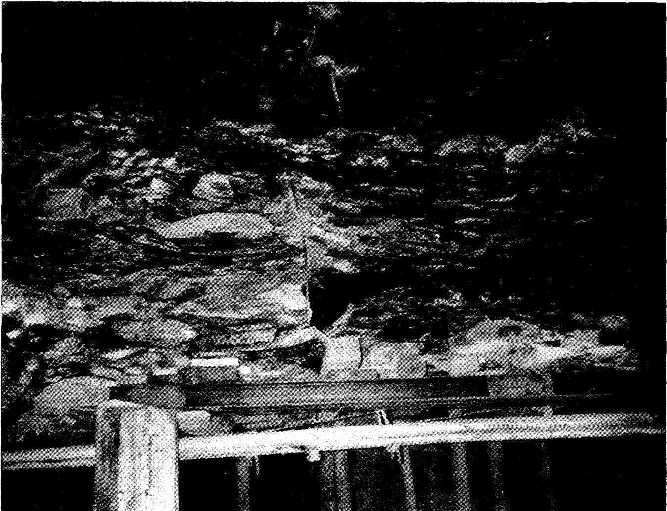
Channel margin roof in Star Point No. 2 Mine. About 2.5 m (8 ft) of interbedded siltstone-mudstone immediate roof has fallen, exposing bottom surface of overlying channel sandstone (dark area surrounding rectangular roof bolt plate).
