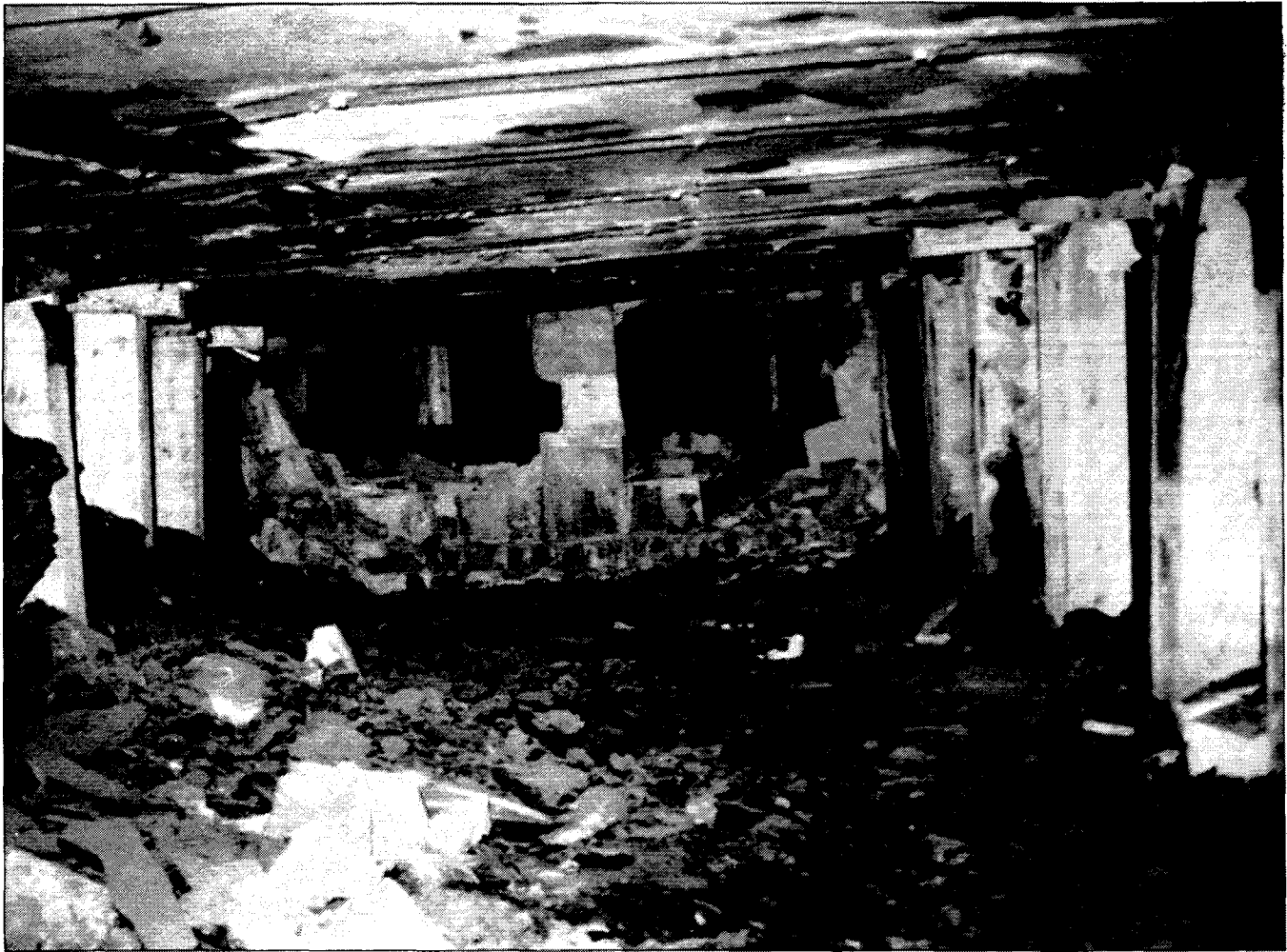
Aftermath of tailgate pillar bump in 8th East gate road. The bump, which occurred outby approaching 9th East panel face, partially filled crosscut with coal thrown from pillars at either side and destroyed solid concrete block stopping.
