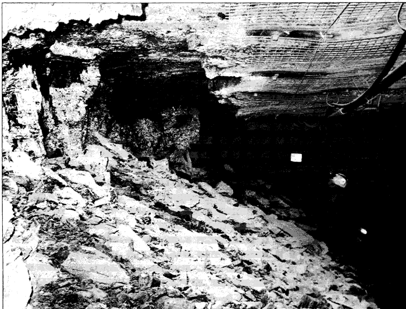
Sloughed rib in Sunnyside No. 1 Mine gate road. Original rib line is seen at roof brow to left of wire mesh. Upper portion of composite seam has fractured and fallen away from roof, covering relatively intact lower part of seam with loose coal.
