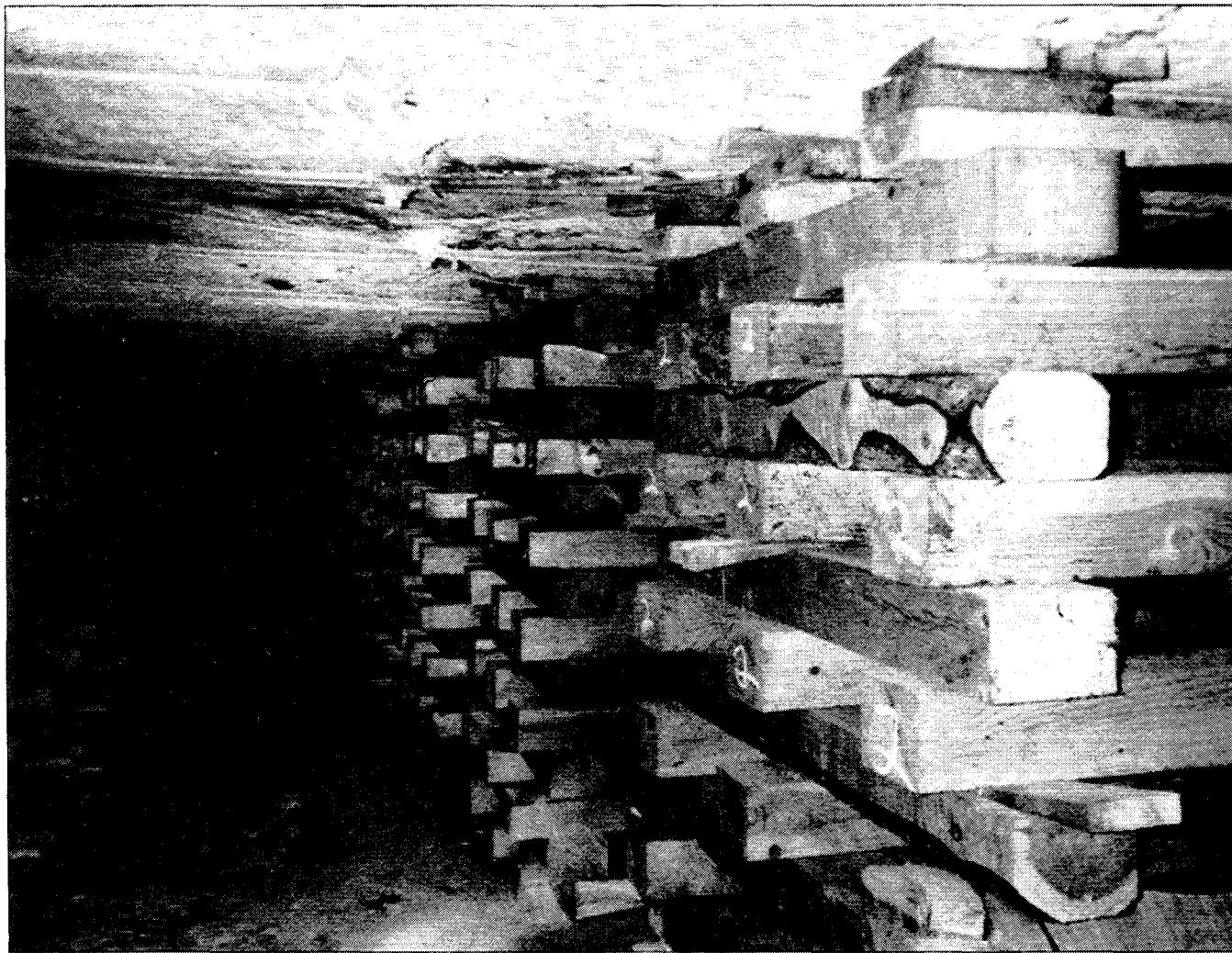
Nine-point cribbing used for secondary support in subsequent gate roads of Star Point No. 2 Mine.
