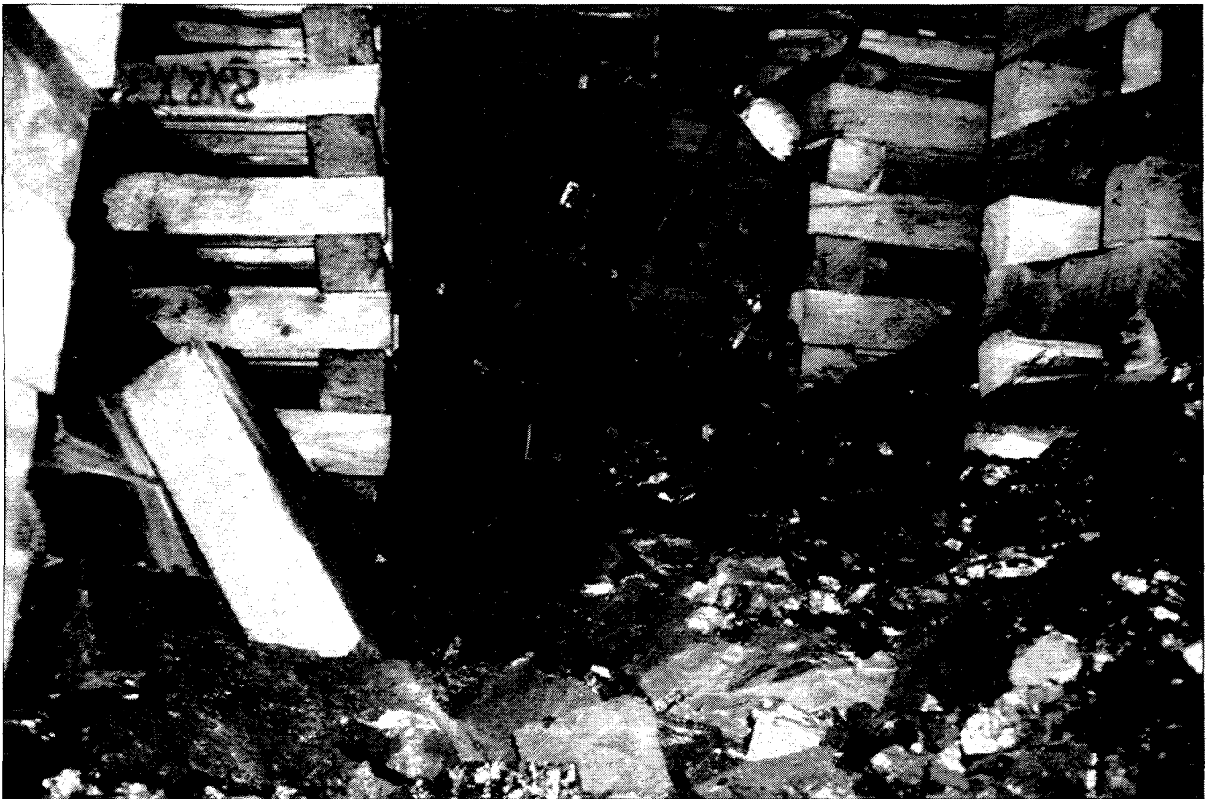
Aftermath of gate road chain pillar bump in northeast part of Sunnyside No. 1 Mine. Crosscut has been mostly filled with loose coal thrown from pillars during bump. Pillars were oversized at 16.8 m (55 ft) wide owing to headgate entry misalignment.
