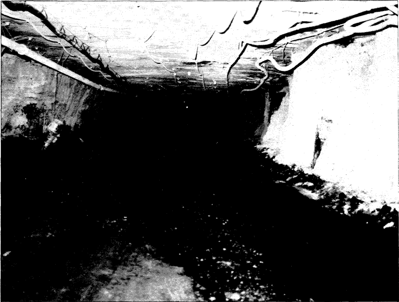
Intake entry of 9th East gate road. Even, unfractured ribs are typical of gate road conditions before approach of 9th East panel face and indicate minimal pillar yielding.
