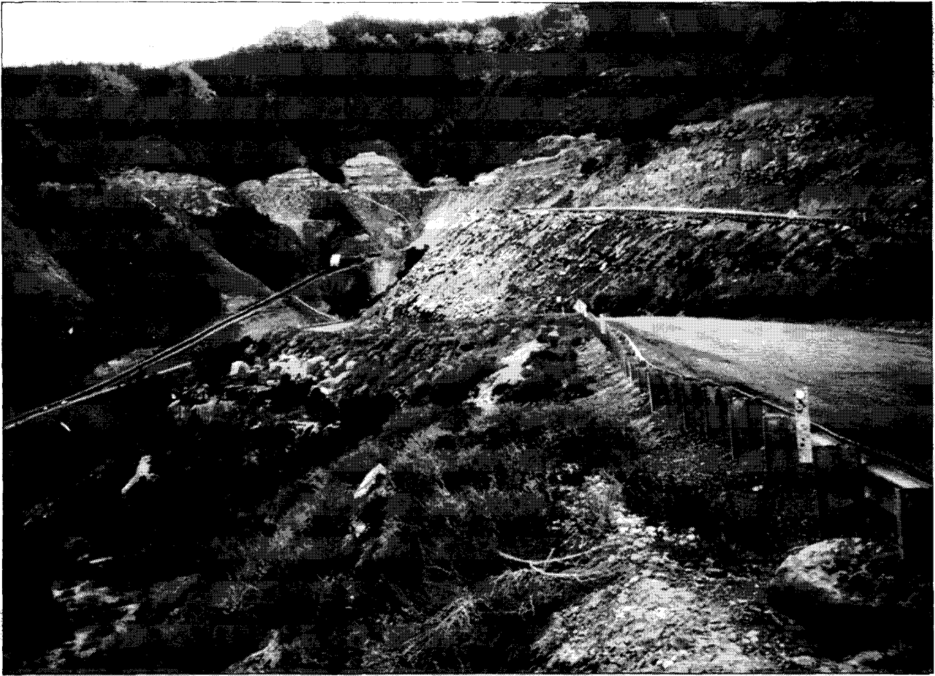
Strata at Star Point No. 2 Mine. From canyon bottom (at lower left foreground) upward, Mancos Shale makes up wooded slope extending up to foot of low cliff and ledge formed by Star Point Sandstone (to left of mine road in foreground). Mine portals in Wattis Seam (in Blackhawk Formation) are at level of bench cut across face of high ridge in background. Blackhawk Formation extends upward to foot of Castlegate Sandstone cliff at crest of ridge.
