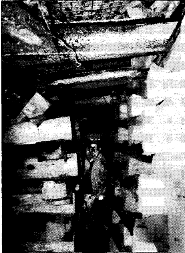
Sixth Left tailgate escapeway during panel 4 mining. USBM engineer wedged between cribs indicates narrow width of escape walkway.
