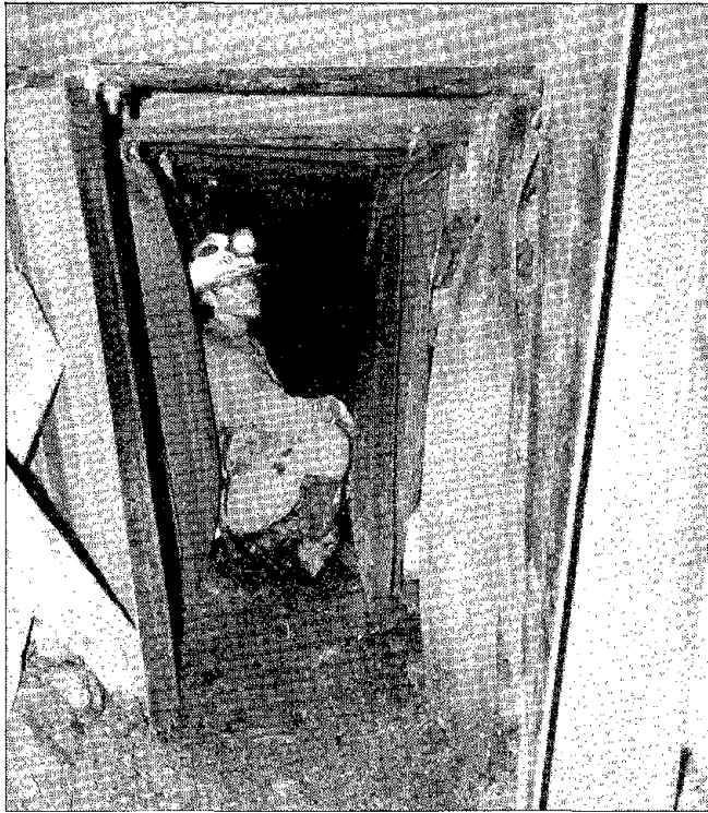
Figure 12.—Additional example of tailgate support requirements when critical pillar is used.
