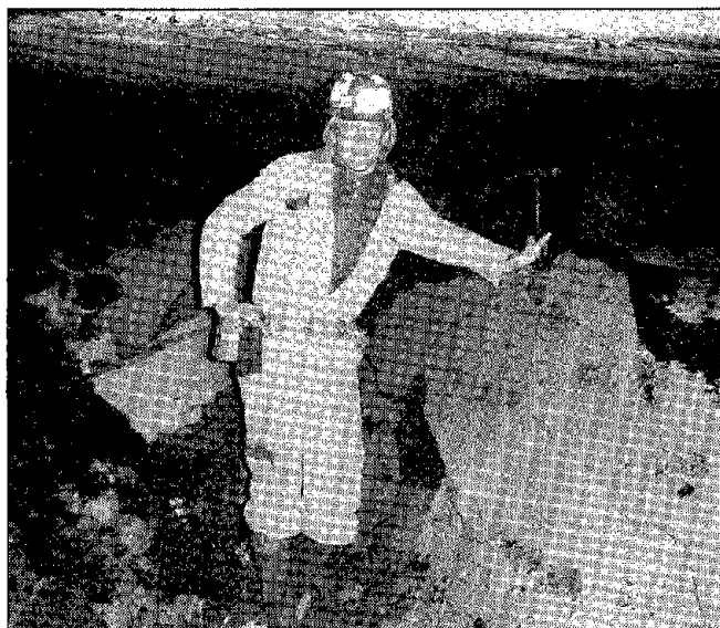
Figure 6.—Severe floor heave resulting from improper pillar design.
