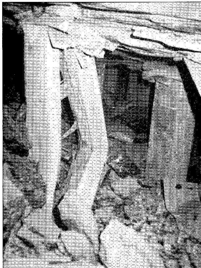
Figure 9.—Critical pillar bump near the headgate corner.
