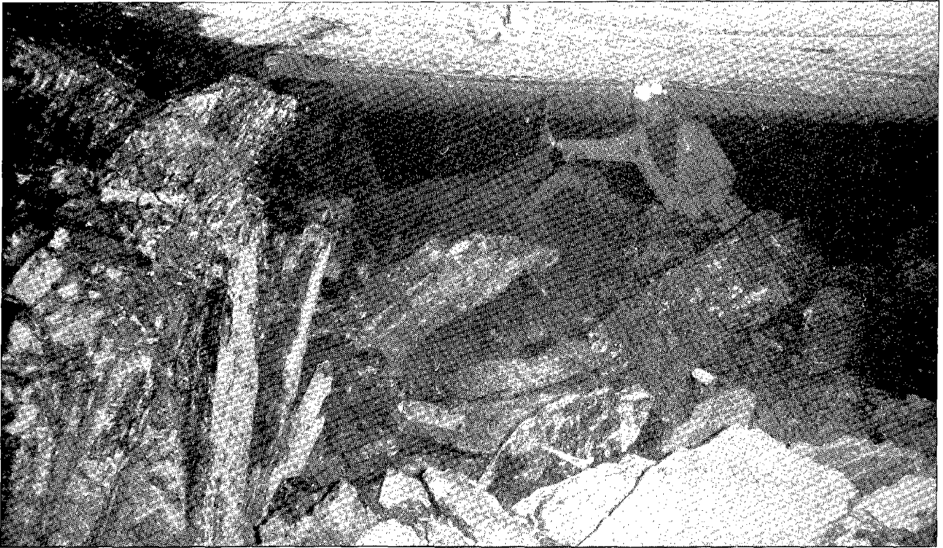
Figure 10.—Severe rib failures accompanying floor heave conditions in a critical pillar application.
