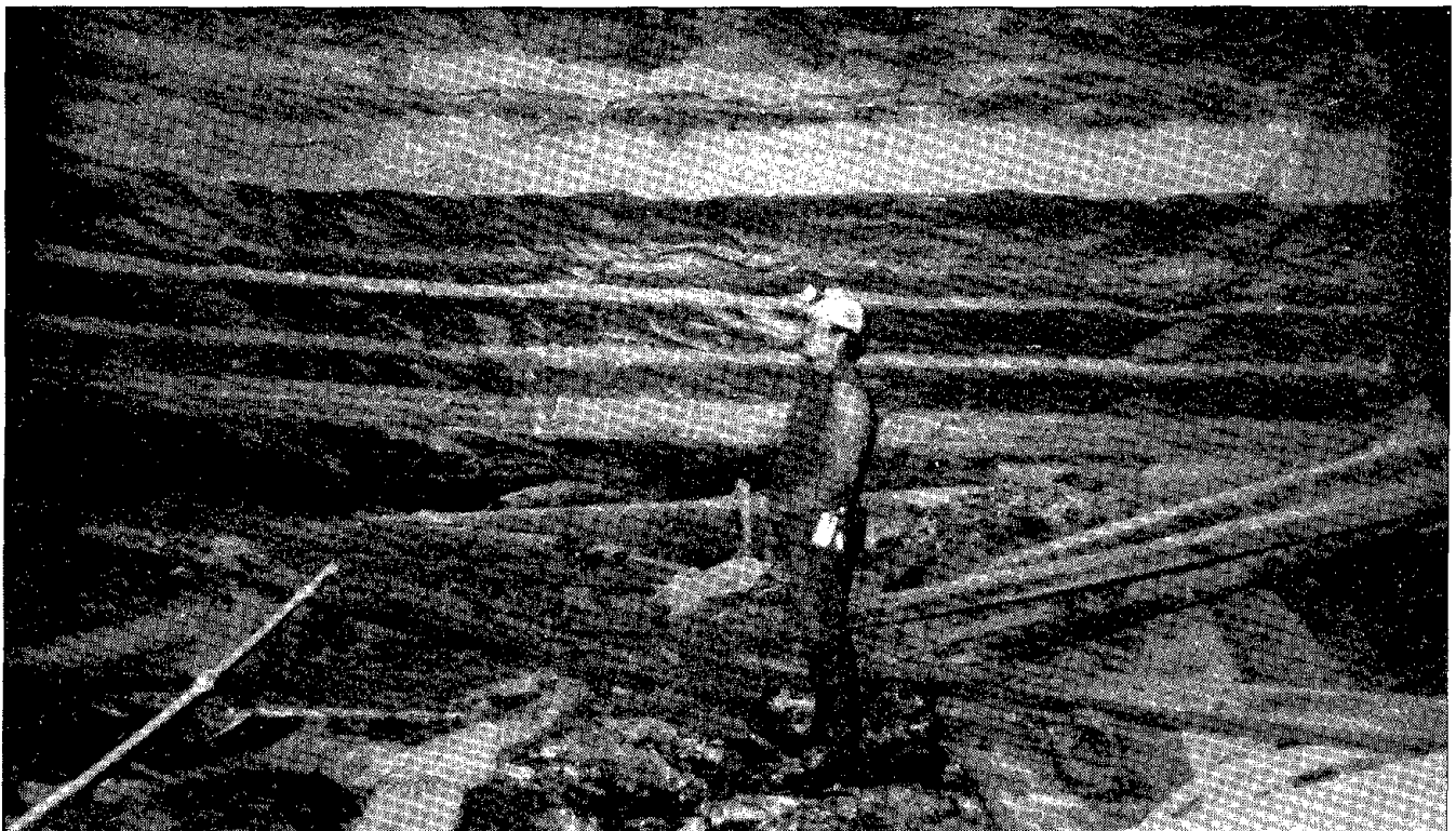
Figure 2.—Typical strong roof strata sequence, found in many western U.S. mines, comprised of fine-grained sandstones, siltstones, and strong mudstones.
