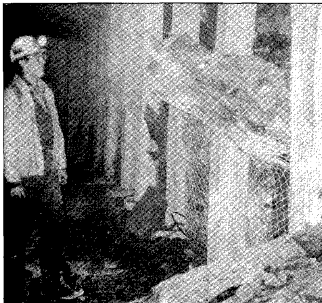
Figure 17.—Although generally successful in controlling rib sloughage, fencing methods must account for rib toppling in high seams.
