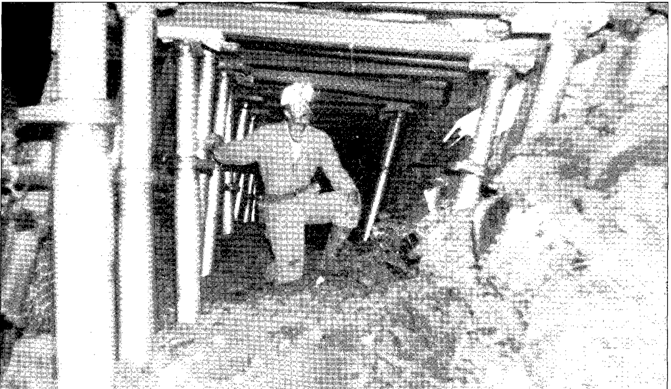
Figure 11.—Intensive mine roof support used to control entry closure in a critical pillar tailgate setting.
