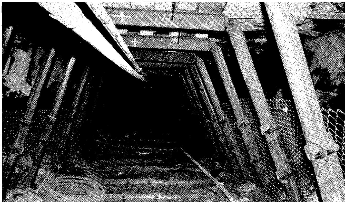
Figure 15.—Steel-set support system, which is no longer used except in the most severe conditions.
