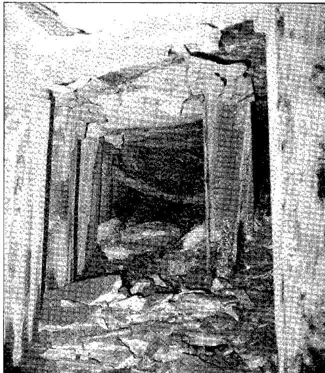
Figure 5.—Poorly laminated, minimally supported mine roof typically cannot withstand the deformations of yielding gate designs.
