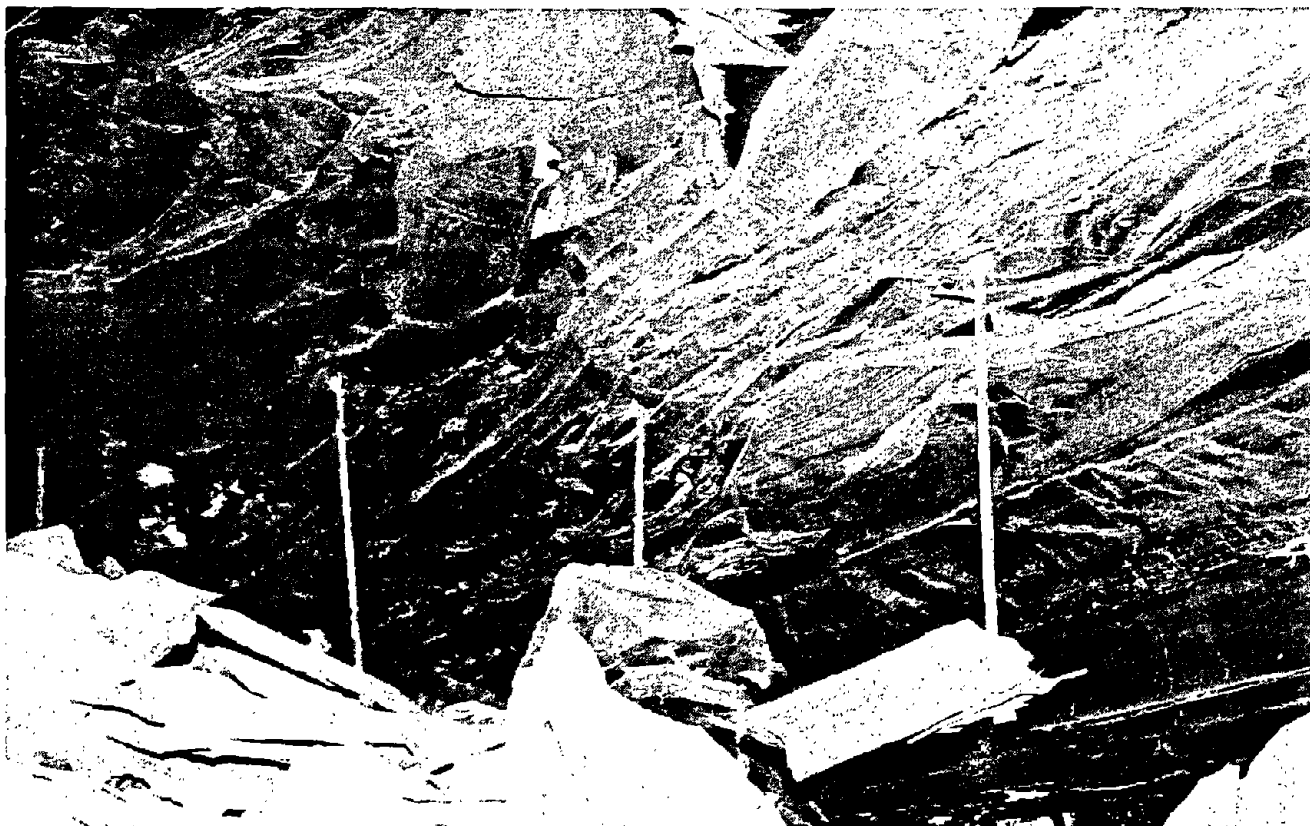
Figure 3.—Weak bedding in a laminated shale.
