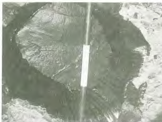
Figure 14.—Slickensided kettlebottom roof void.
