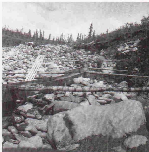
FIGURE 6. - Gold sluicing operation on Valdez Creek, circa 1915 (photo courtesy of the U.S. Geological Survey).
