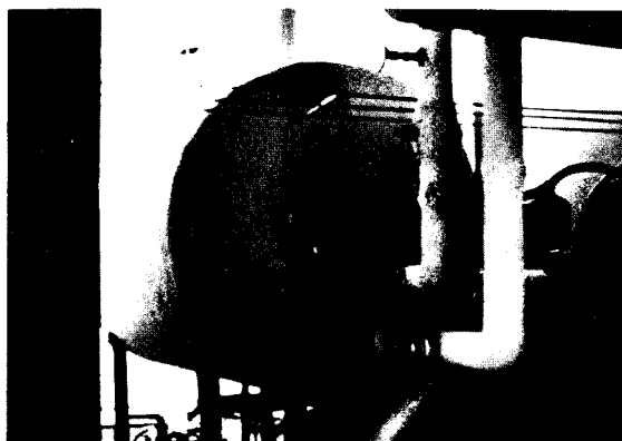
FIGURE 12. - Domestic hot water being heated by geothermal water at Oregon Technical Institute (Klamath Falls, Oreg.).
