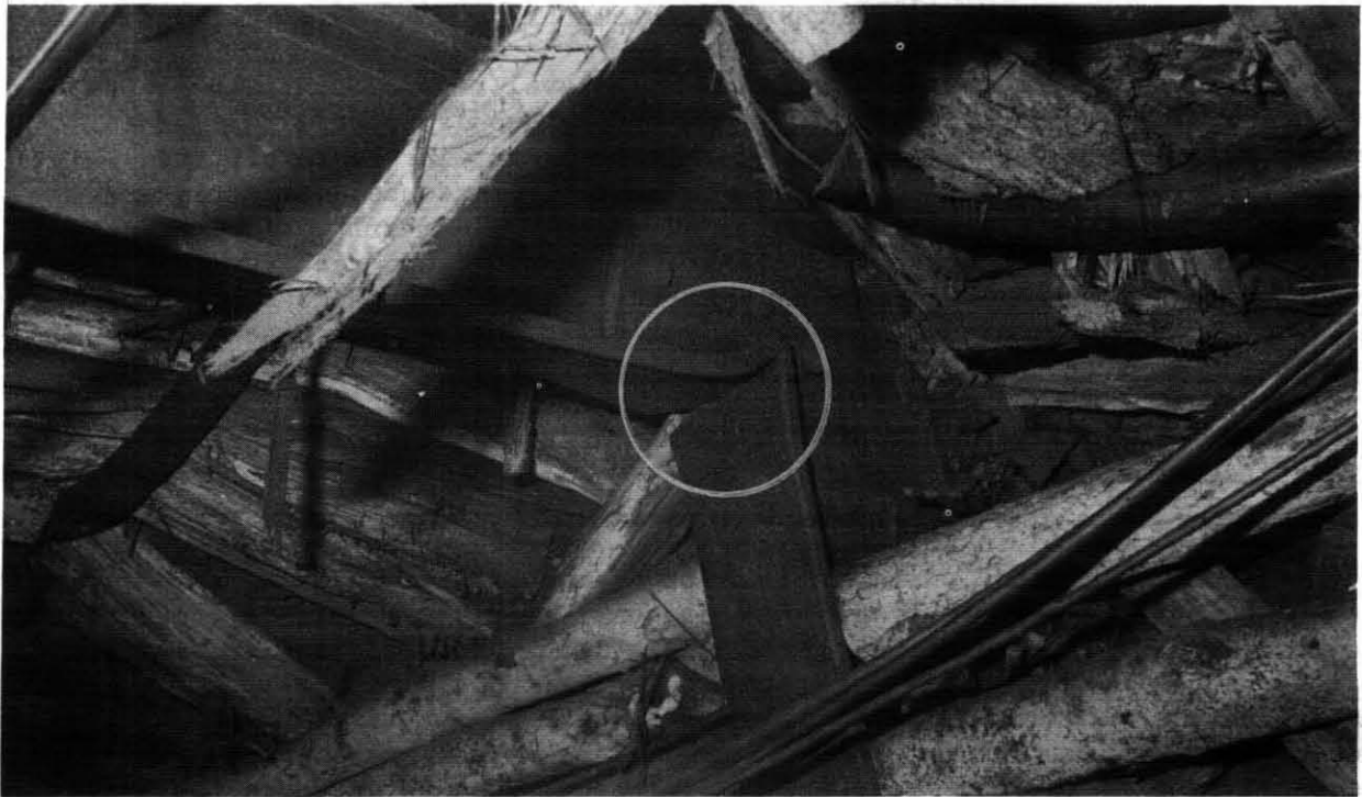
FIGURE 15. - Common distortion of sets. Note pipe spiling at upper right.
