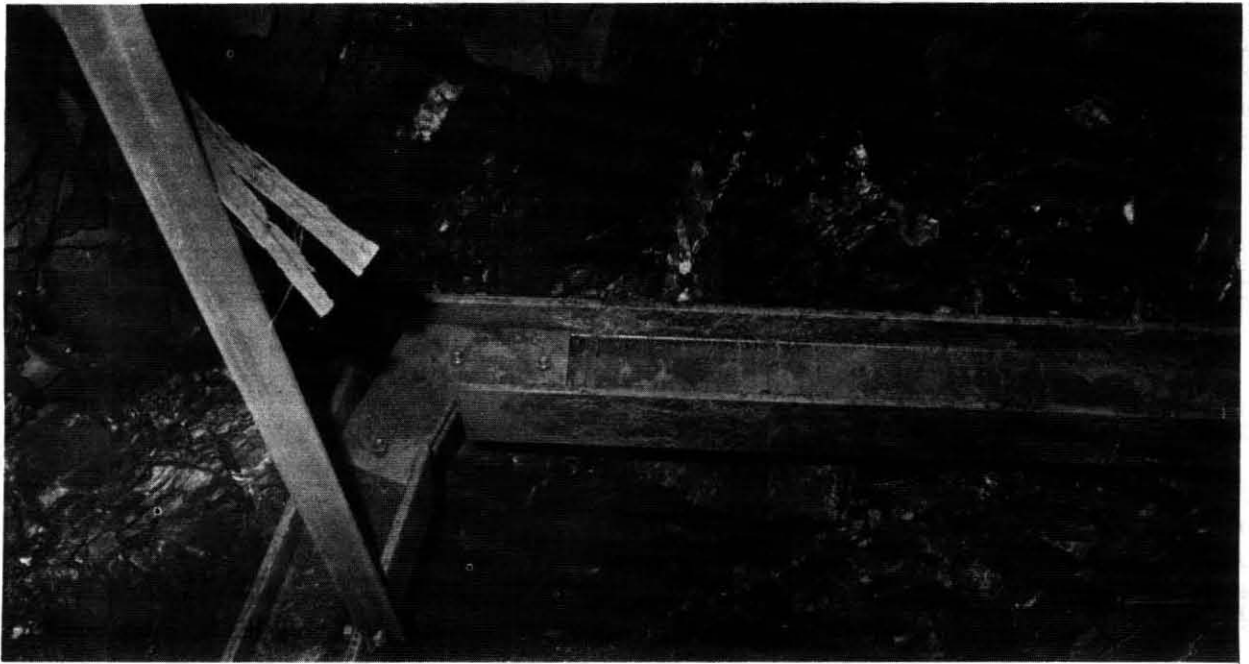
FIGURE 13. - Fifty-eight-pound wide-flange steel set in position prior to final assembly of post and cap.
