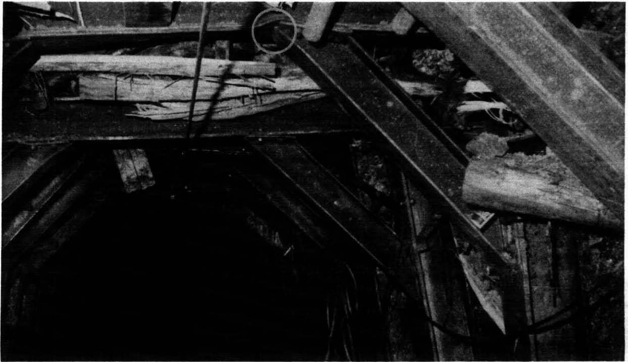
FIGURE 19. - Local deformation at ends of knee braces.
