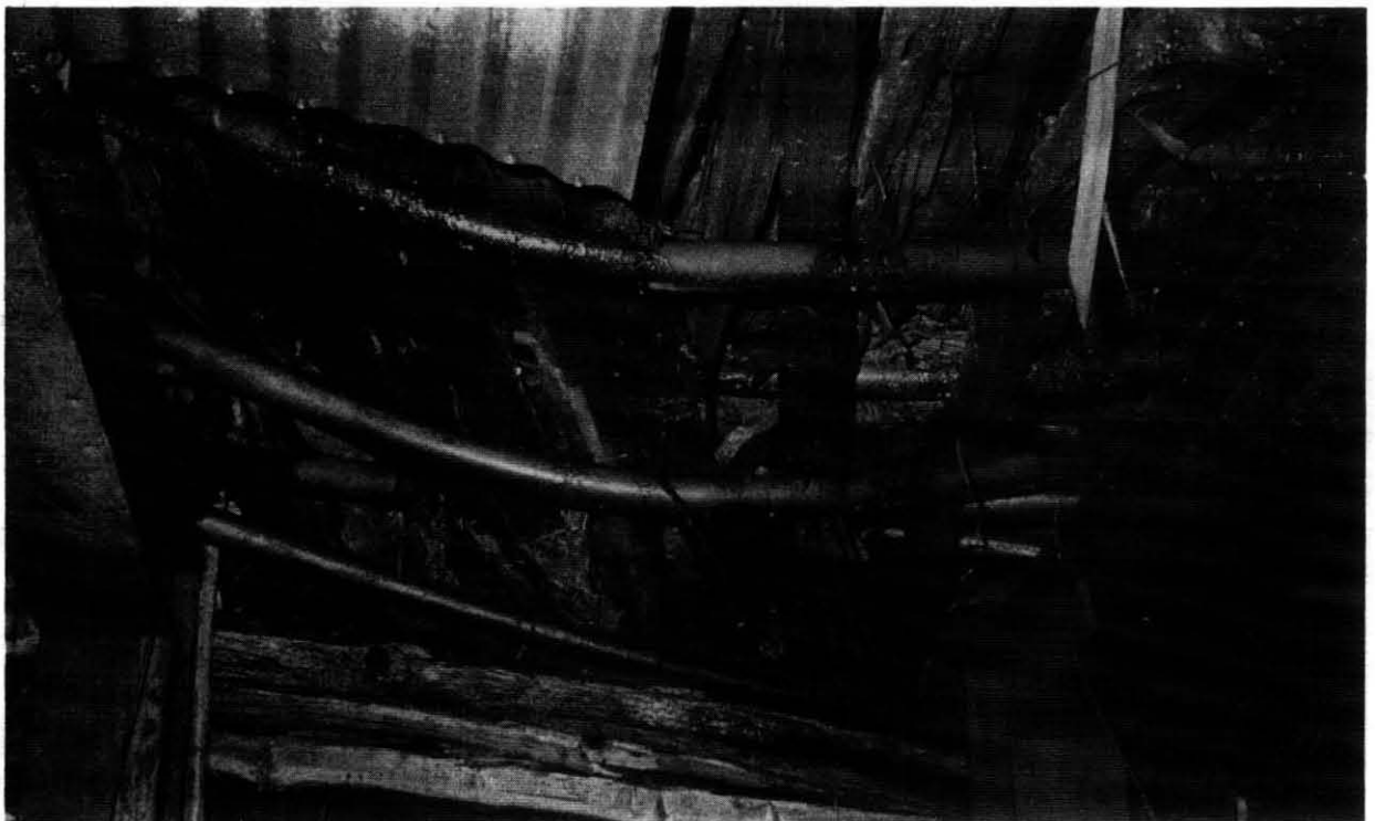
FIGURE 10. - Crosscut sets with yielding of sets apparent.
