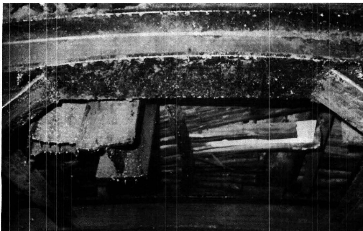
FIGURE 18. - Bending up of cap due to side pressure.
