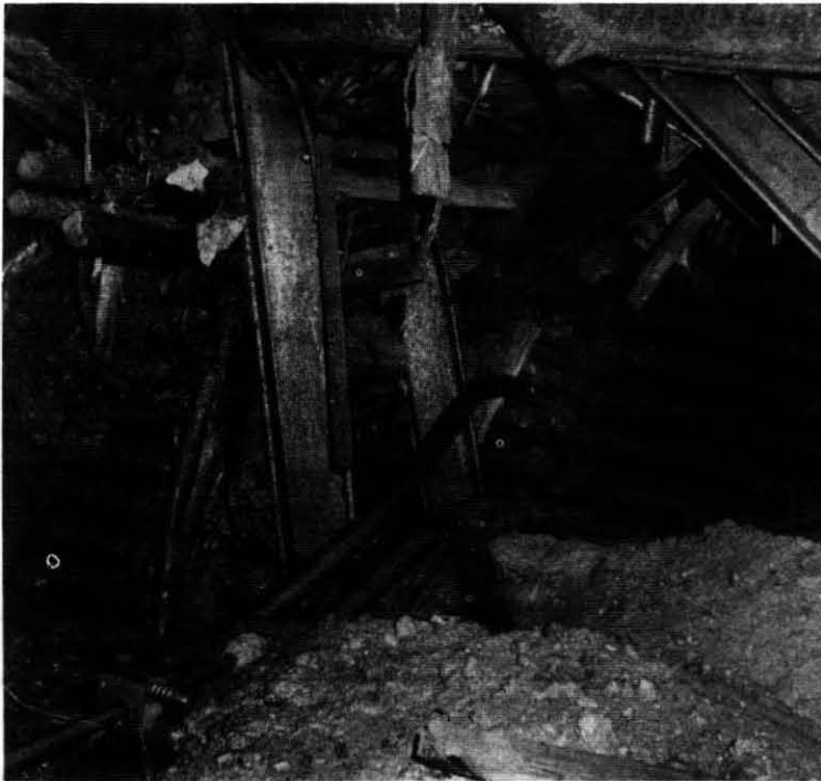
FIGURE 24. - Left rib of crosscut shown in figure 23. New post visible in left foreground.
