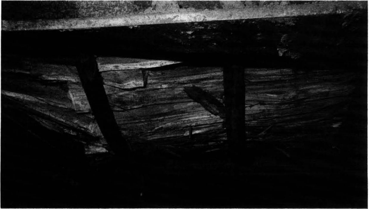
FIGURE 9. - Crosscut sets showing distortion of sets and "basket" effect of back spiling.
