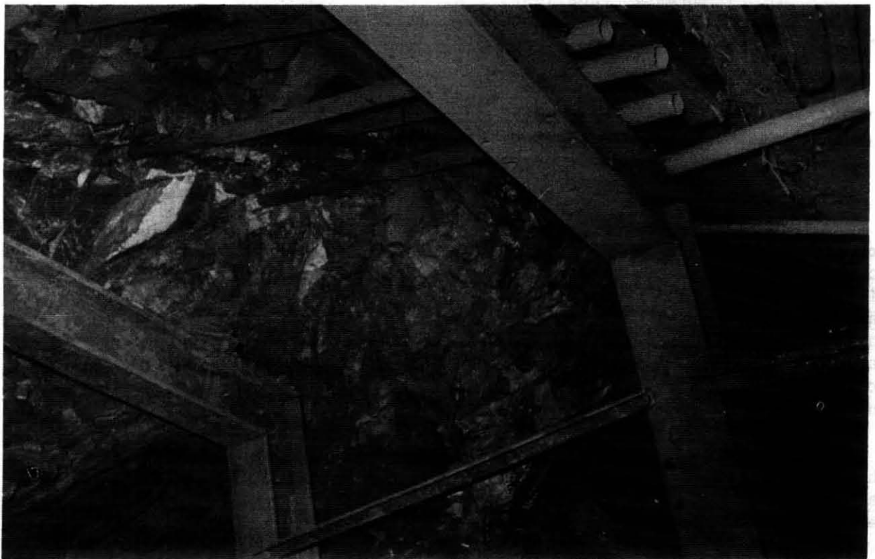
FIGURE 14. - Right-hand corner of set shown in figure 13. Vertical misalignment is due to intentional lowering of track grade at this particular point.
