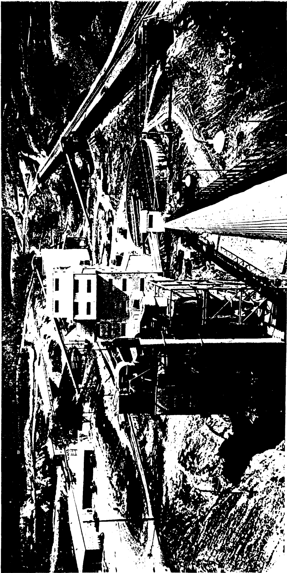
At this modern West Virginia coal preparation plant, coal is crushed, cleaned, washed, and dried before being shipped to
